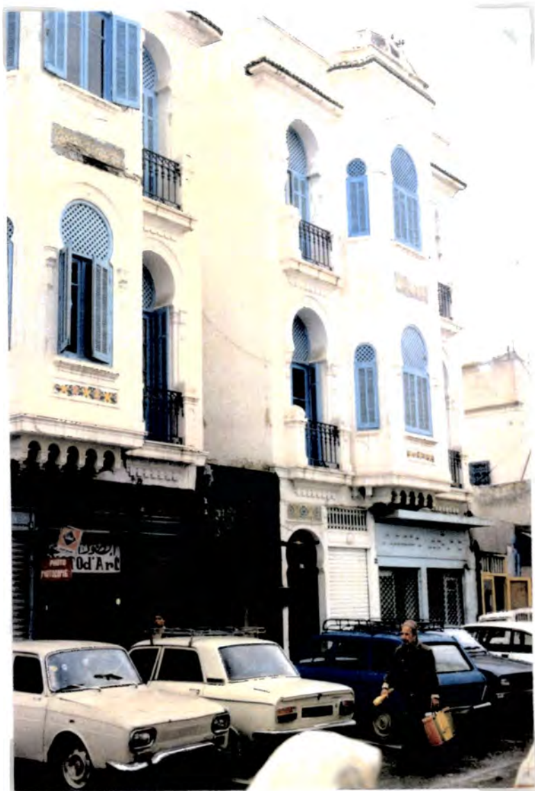
Plate 15: Turn of the century building in the style arabisant at Bab Souika. Photo taken January 1991
