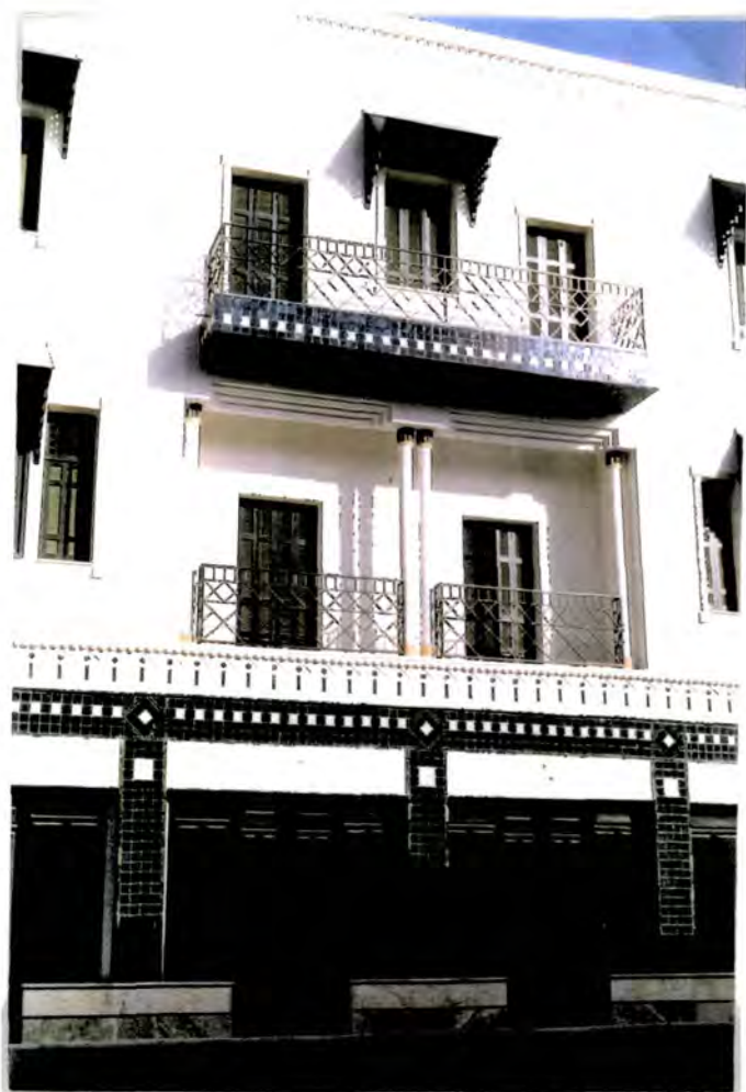
Plate 28: Bab Souika urban renewal area: apartment buildings on the Rue Bab Benat by T. Ben Miled and M. Ridane in a reworking of the style arabisant.
