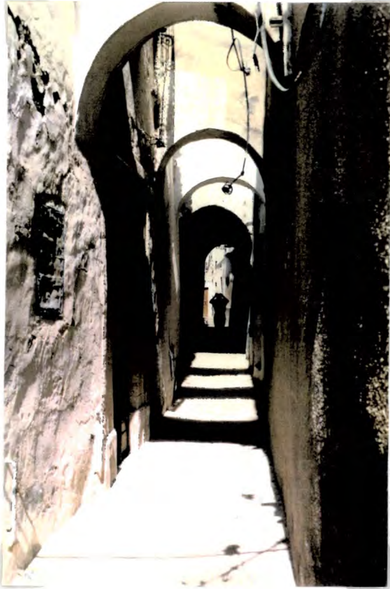
Plate 3: a zanka, a narrow alley in the Medina, partly covered by extensions to the houses either side constructed over the street.
