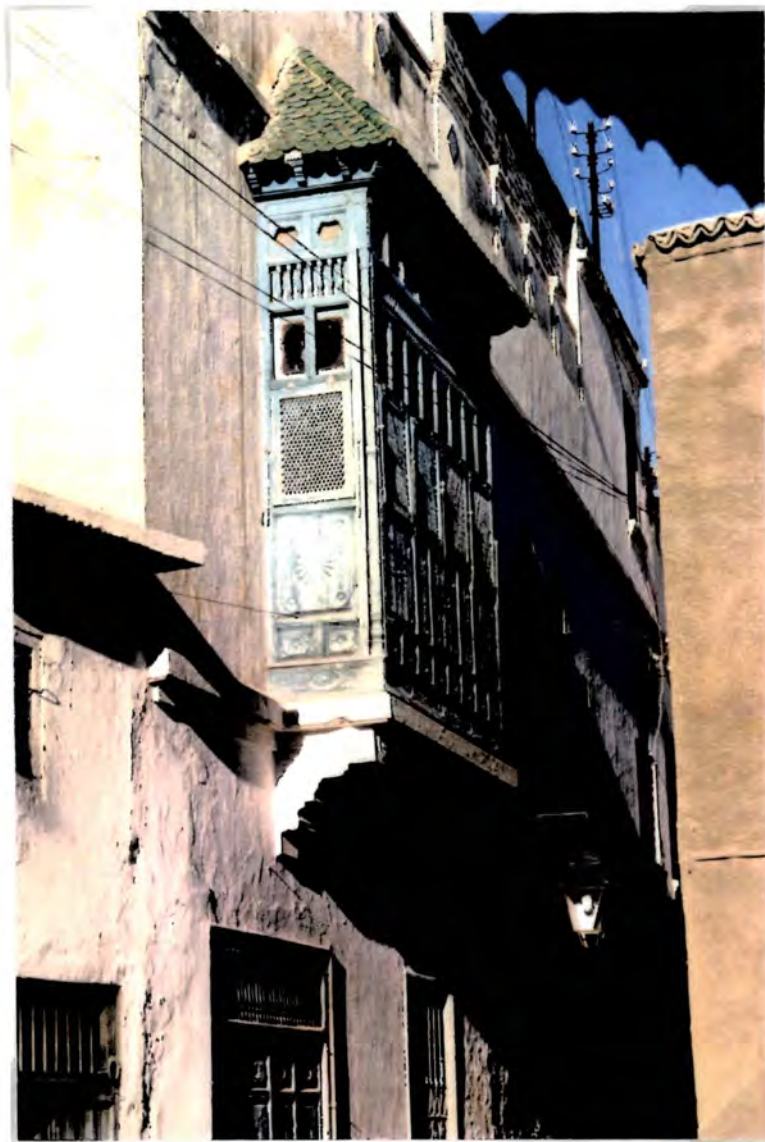
Plate 5: a GANERIA, the Tunisian covered balcony. The wooden superstructure could be very elaborate, including lattice work wooden shutters and coloured glass in some of the windows.
