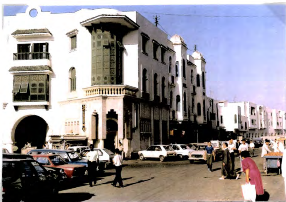
Plate 17: The new post office at Bab Souika, completed May 1987
