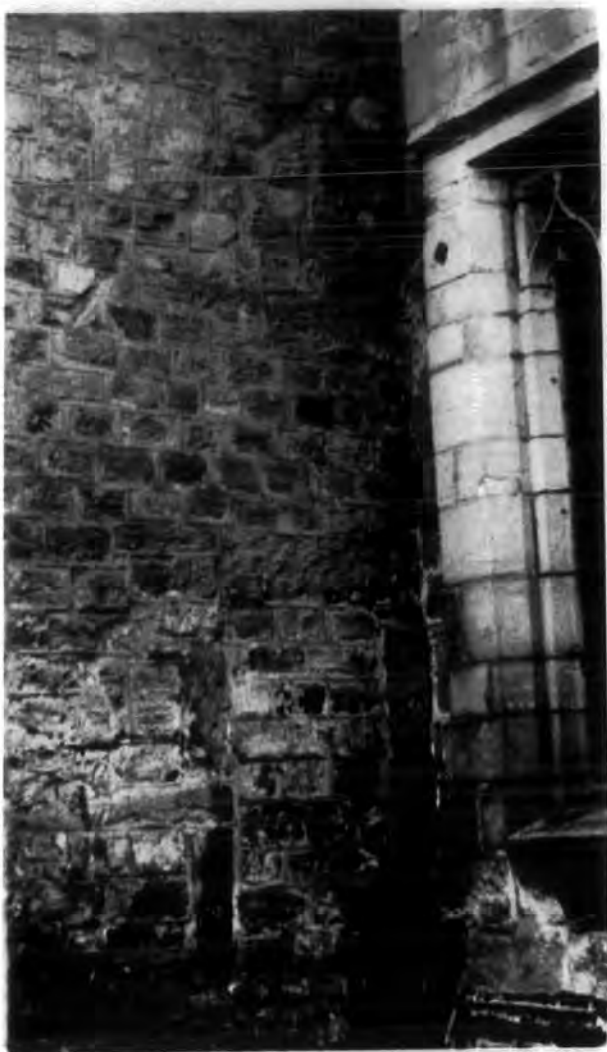
ST PETER North porticus: gable line and doorway
