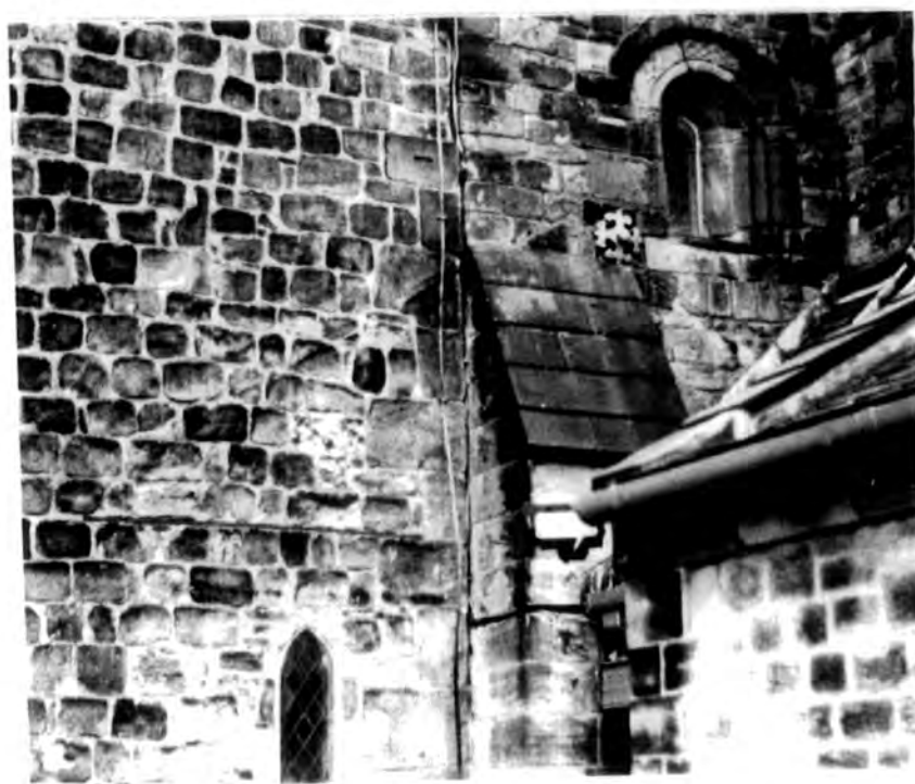
North wall: tower window and gable lines
