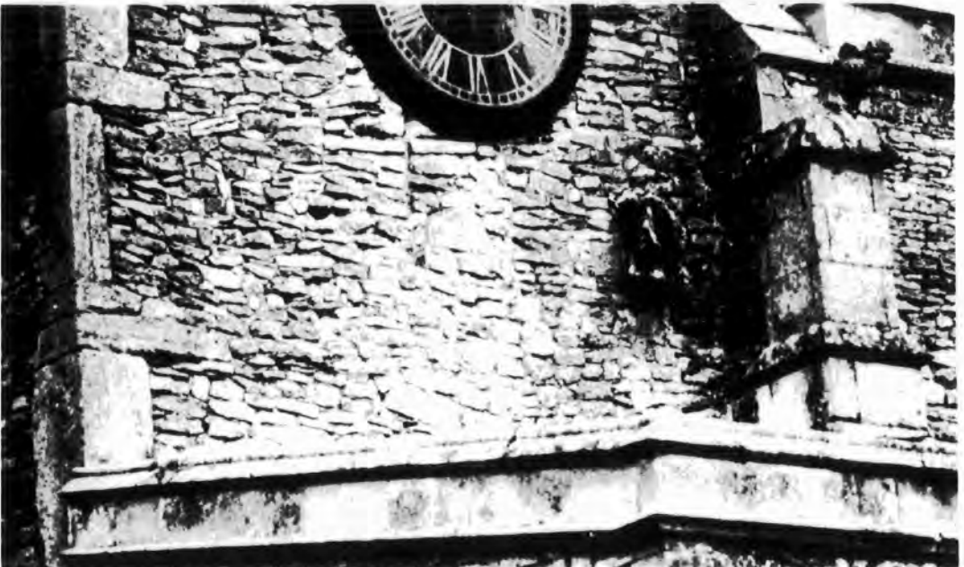
Detail of tower's south face: blocked opening
