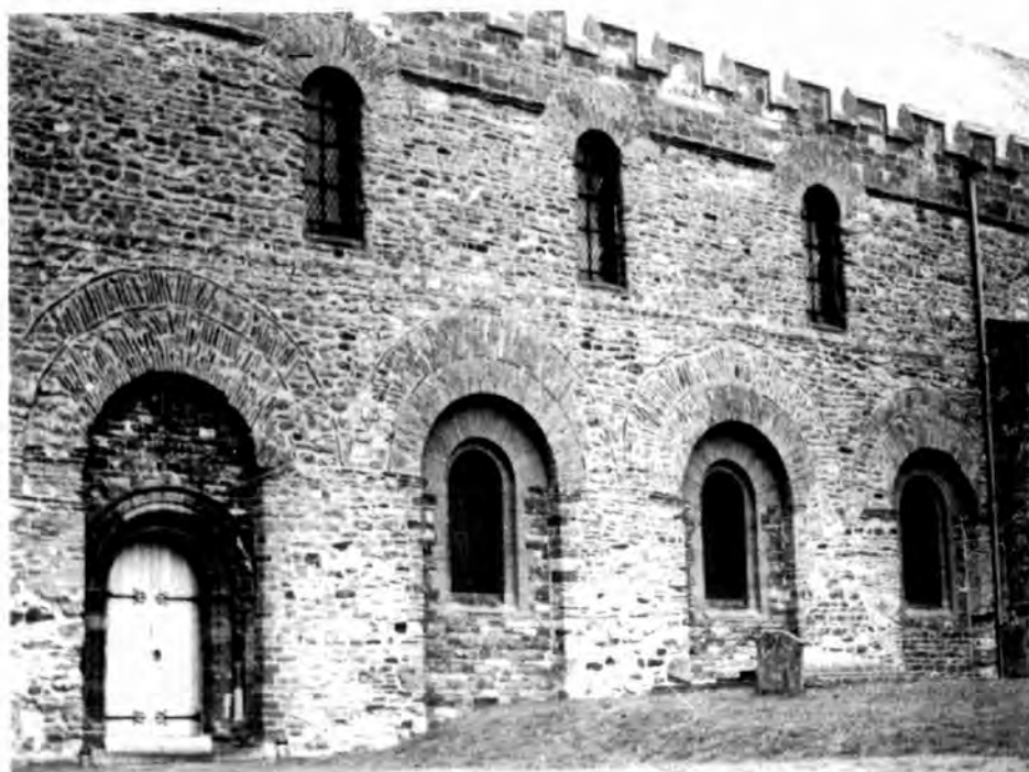
South wall of nave
