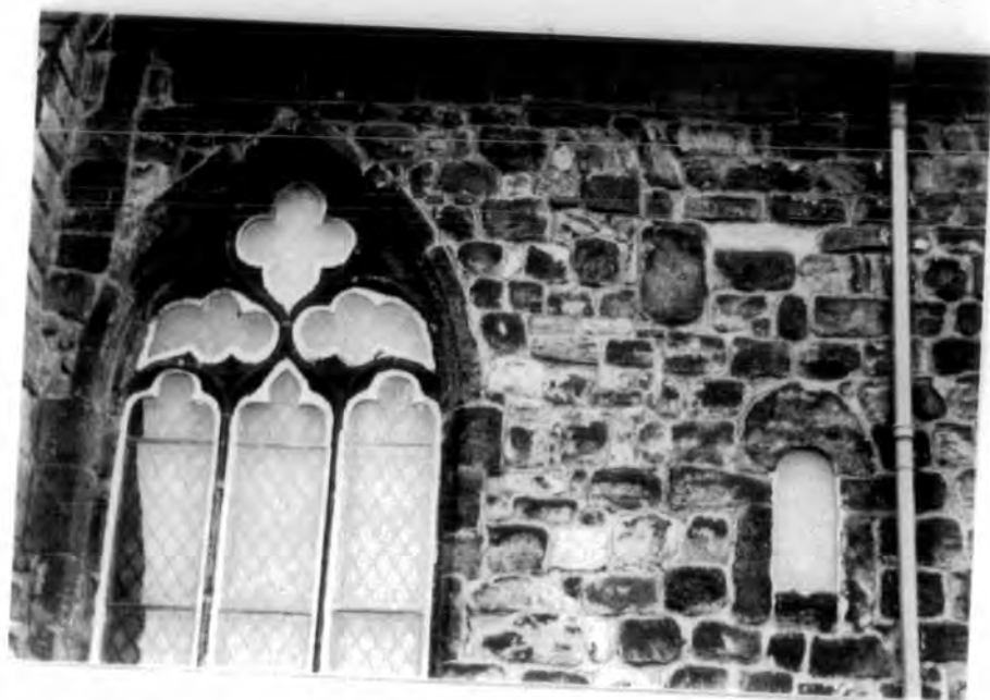
South wall exterior: upper doorway
