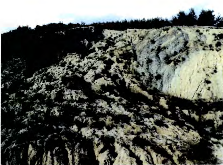
photograph 3.6 Part of the Krevatina failure at location KVT 1.
