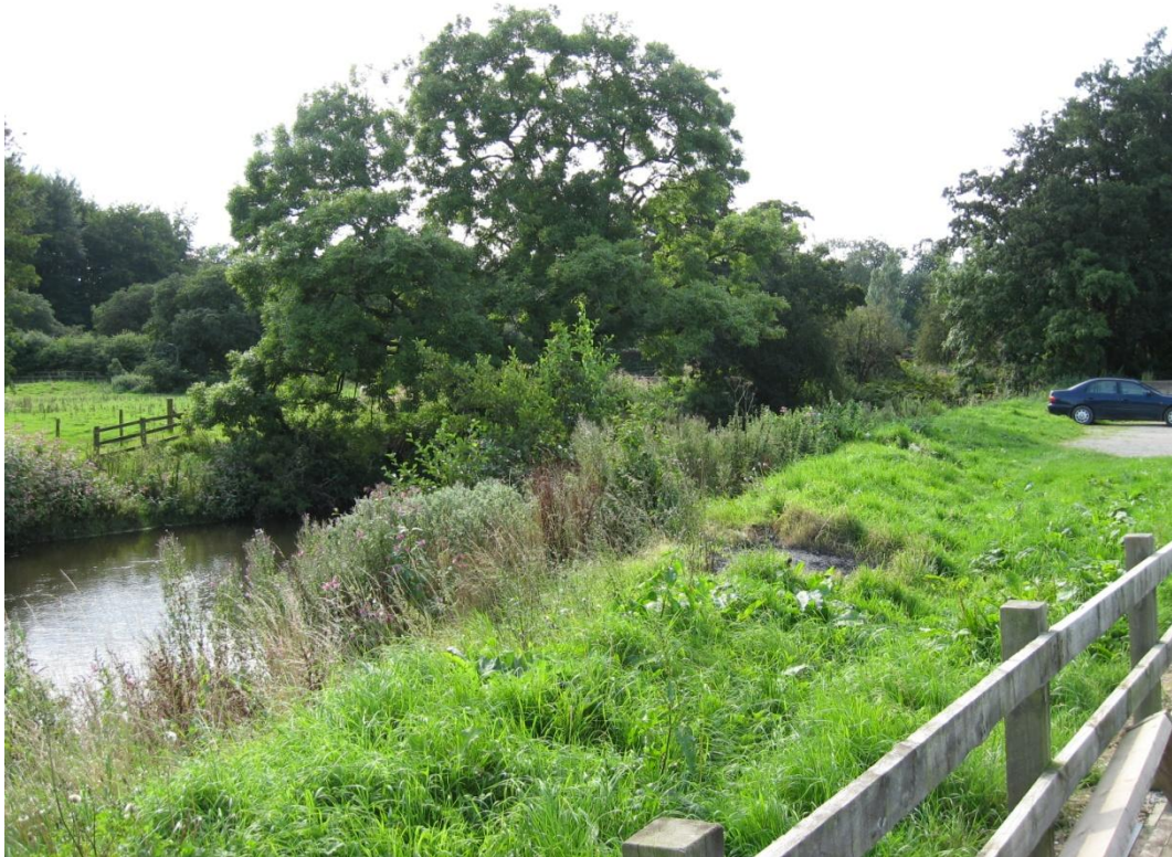
Figure 5.4: The raised river bank of the River Rye, work completed prior to the 2005 flash flood, built between the River Rye and the houses in Bridge Farm Close and Ryegate in Helmsley.
