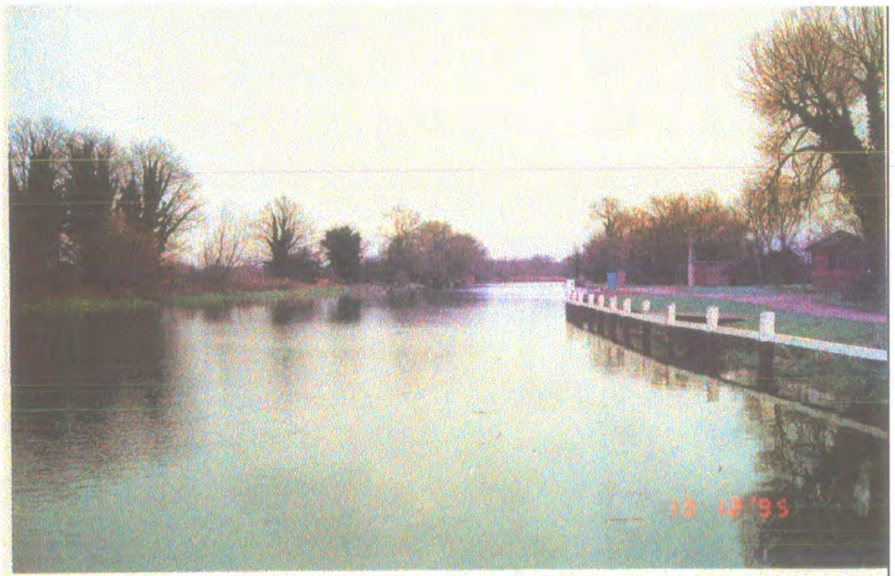
View from sampling site looking upstream
