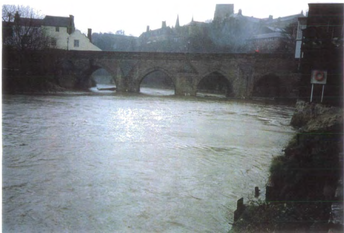
Plate (3.5) The Old Elvet Bridge
