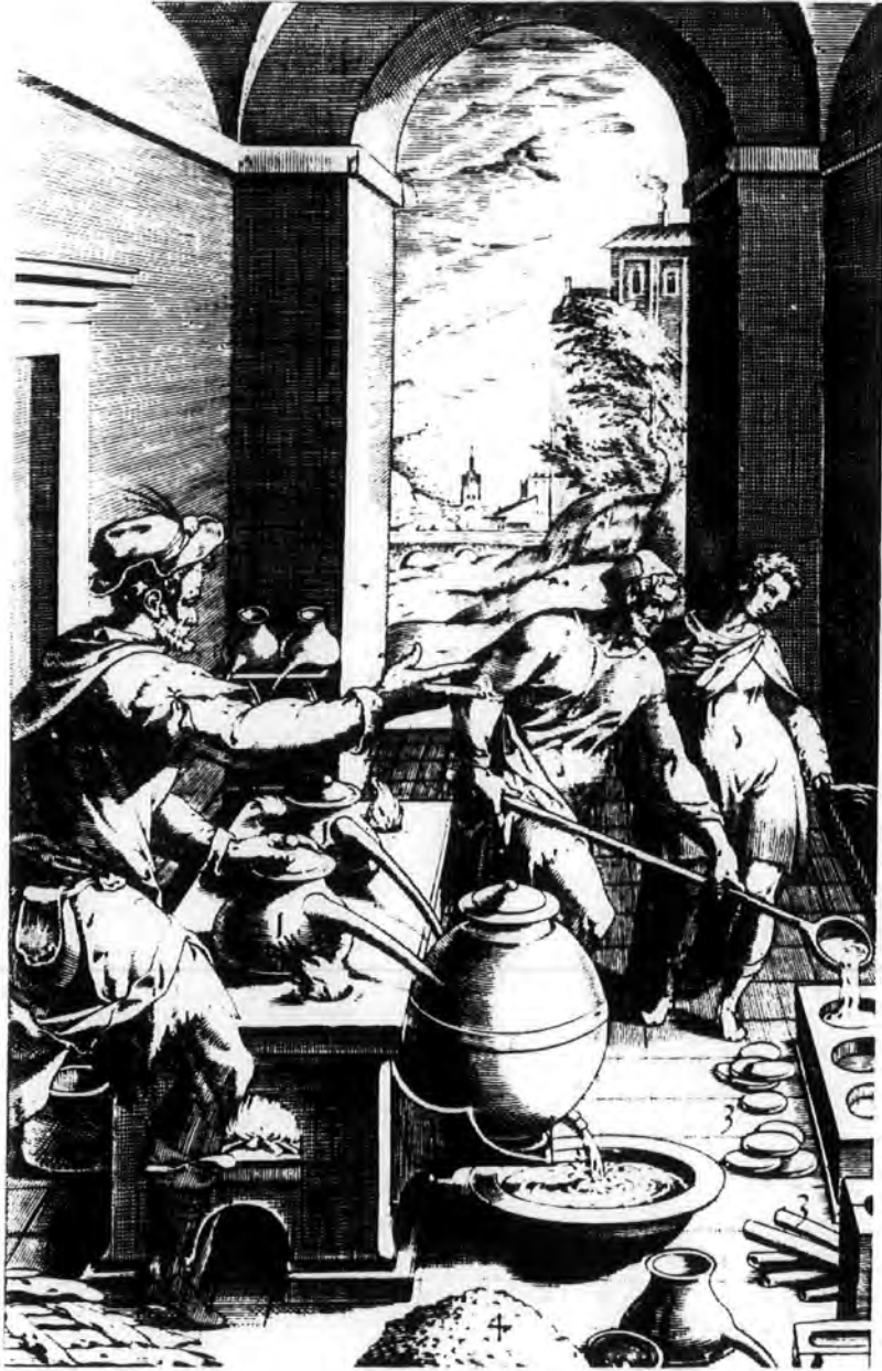
V DISTILLATION OF SULPHUR From M. Mercati. Metallotheca , Rome, 1719, p. 78
