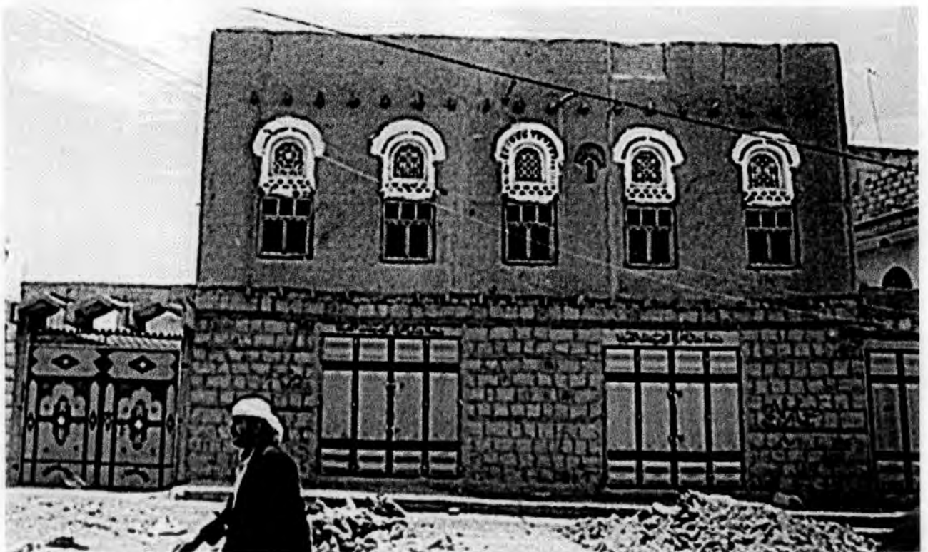
Top and centre - Plans of demonstration house in libn , Sana'a, and building a mud block arch with flexible steel shuttering, Sana'a, 1972 (source Bertaud:71); bottom - stone and libn building, Rada'; opposite - stone, libn and concrete block, Rada', 1990
