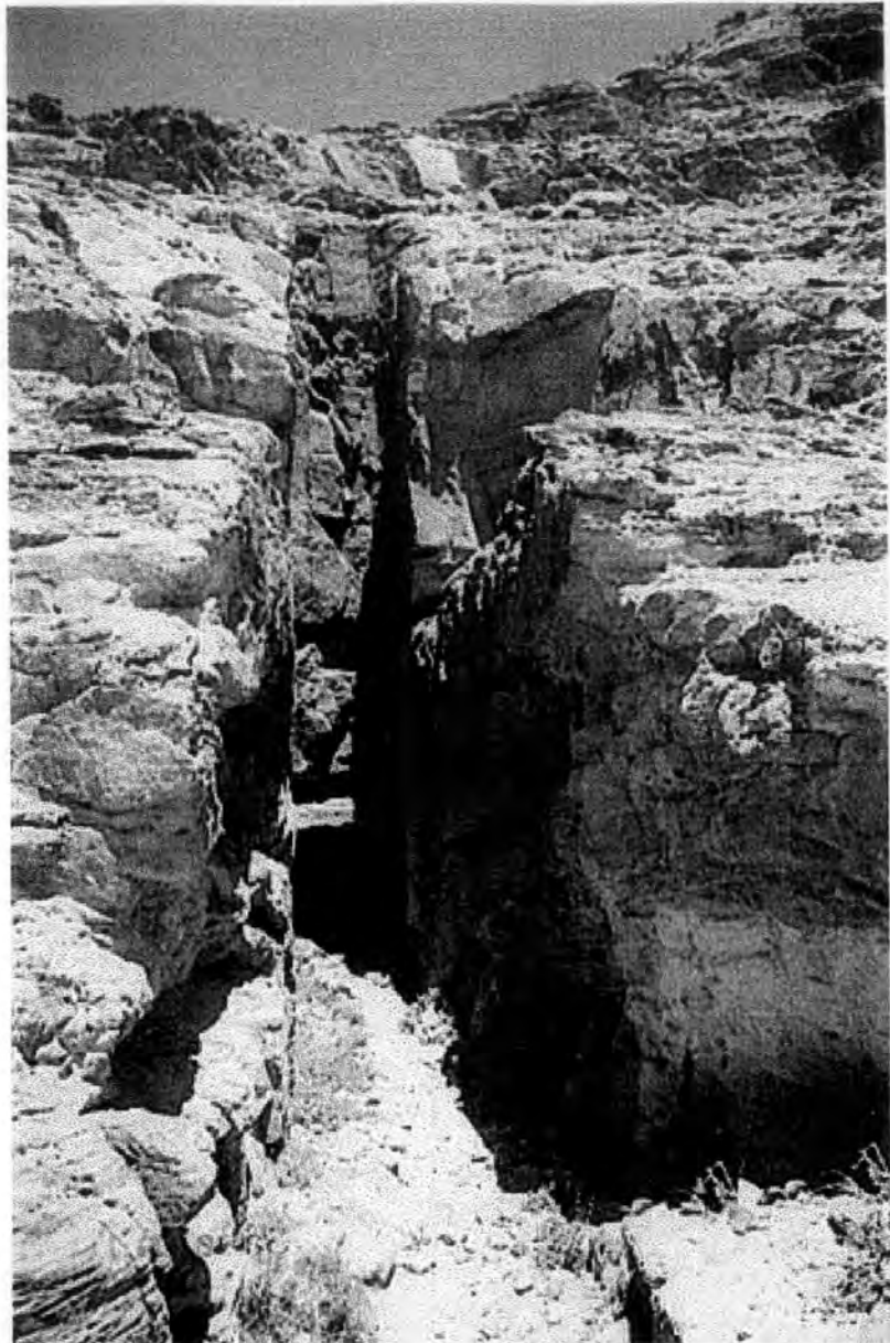
Pre-Islamic irrigation works. Top, left and right - Bainun, Al Hada: canal tunnelling the hill; bottom - The Marib Dam
