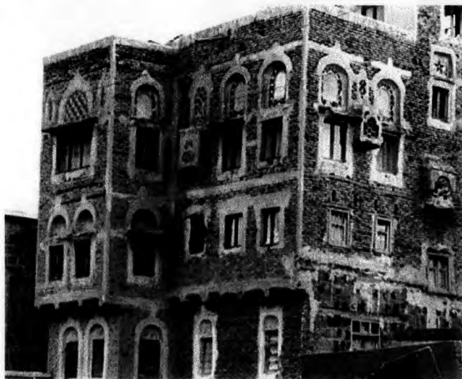
Top - Basut in Ibb (left) and Jubban; centre left - Thula; right - Yarim; bottom - Al Qa'a, Sana'a; opposite - Early 1970's concrete cantilevers in Sana'a (left) and Hodeida (right)
