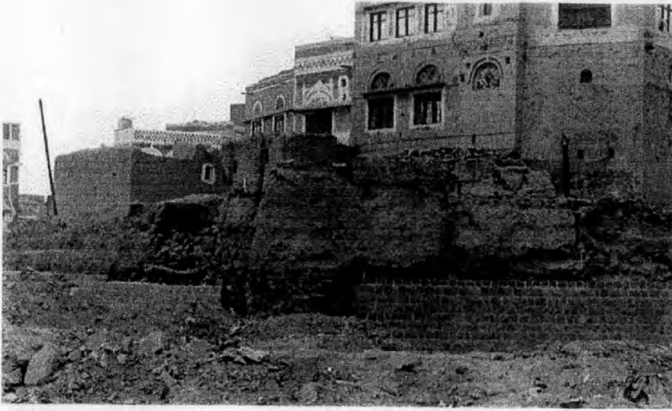
Restoration of the City wall, Sana'a 1990
