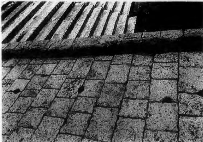
Top - Water tank, part of Dhamar's municipal supply, 1976; centre left - "Water Room" in a Zabid house (photo S. Kennedy); right - Roof tank , Sana'a; bottom left - Holes in the pavement draining rain water onto the sabil, "Maydan" mosque, Hajja; opposite - Fibreglass water tanks at Sana'a ( top and bottom left ) and Sa'da
