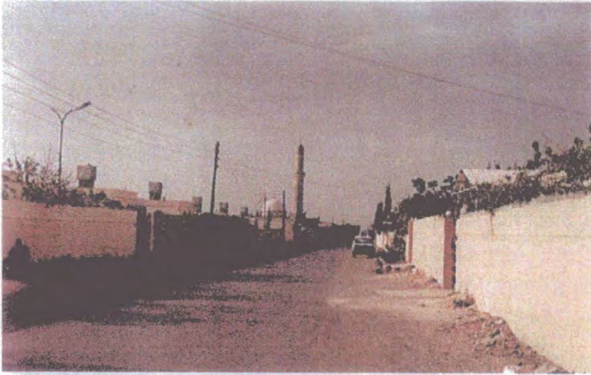
This page - Madina Sakaniya, Sana'a; opposite - Addition of floors to former standard single-storey type, Madina Sakaniya, Sana'a
