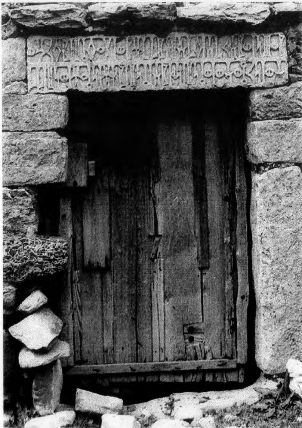
Kawkaban ( top ) and Marib ( bottom ) - pre-Islamic inscription, frieze and other stones reassembled in the construction of later buildings.
