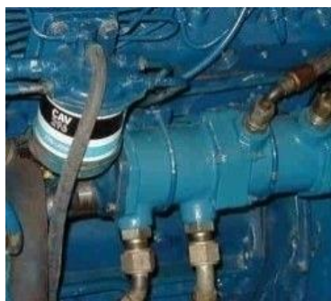
Figure 22: Image of a pump (Source: FLIR Systems, Inc.)
