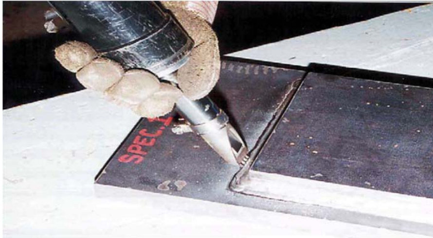
Figure 8: Ultrasonic peening being applied to a steel weld toe [92].
