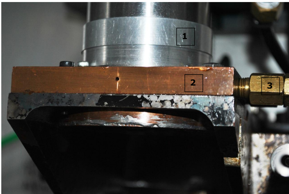
Fig. 3.13. Copper base chiller unit (marked '2') attached to the base of the vertical bearing (marked '1'). Water enters and leaves the unit through pipes connected to the unit (marked '3').
