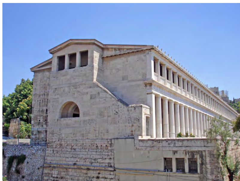
Figure 22. Athens, Stoa of Attalos. Illustrating straight stair at the end of the building. Photographer: A. Babili.
