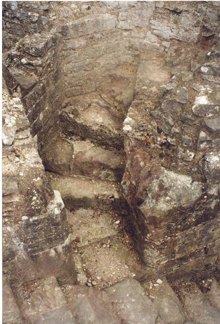
Figure 82. Denbigh Castle: Spiral to the Green Chambers. Illustrating straight steps from the postern with a door off locked from the inside with a drawbar and spiral steps to the Green Chambers. Photographer: C. Ryder.
