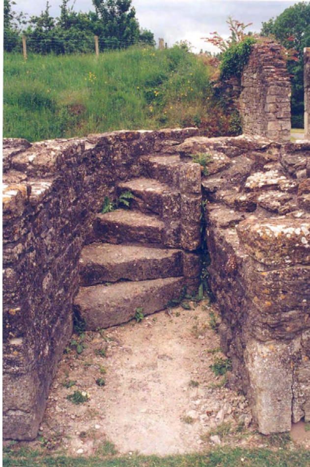
Figure 88. Farleigh Hungerford West Gate. Illustrating the spiral stair to the former accommodation above the West Gate. Photographer: C. Ryder.
