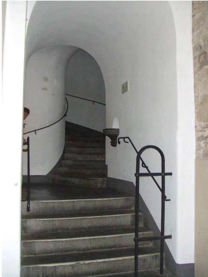
Figure 99. Aachen, Charlemagne's Chapel: Spiral Stair. Illustrating the wide north spiral stair and its vaulting. Photographer: C. Ryder.
