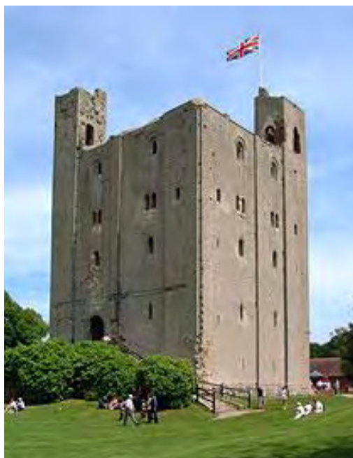
Figure 59. Hedingham Castle Keep. Illustrating first floor entrance and left-hand tower containing the spiral stair. http://www.castlexplorer.co.uk/england .
