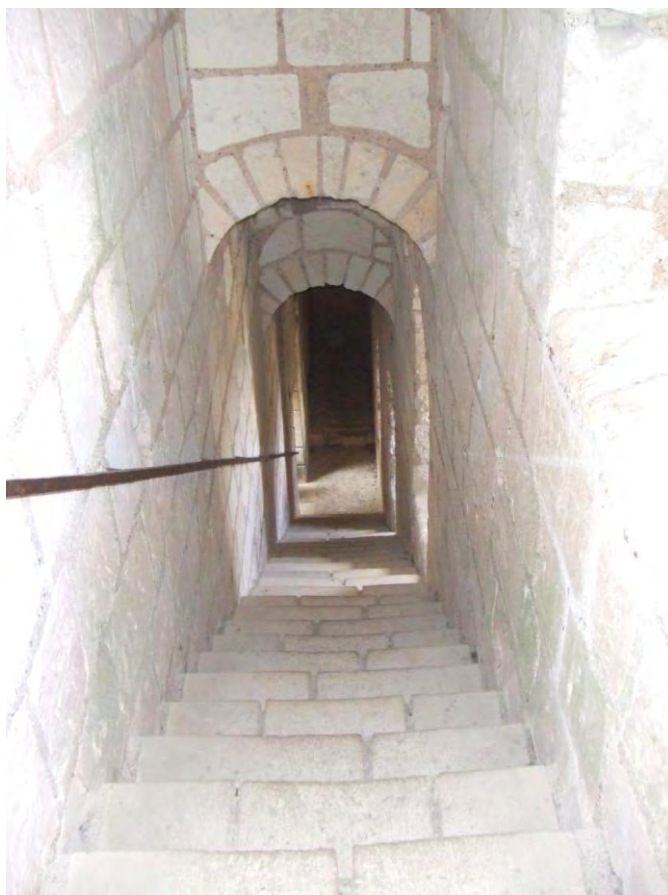
Figure 36. Loches: Interior Straight Stair. View down the interior straight stair in the grosse tour lower levels. Photographer: C. Ryder.
