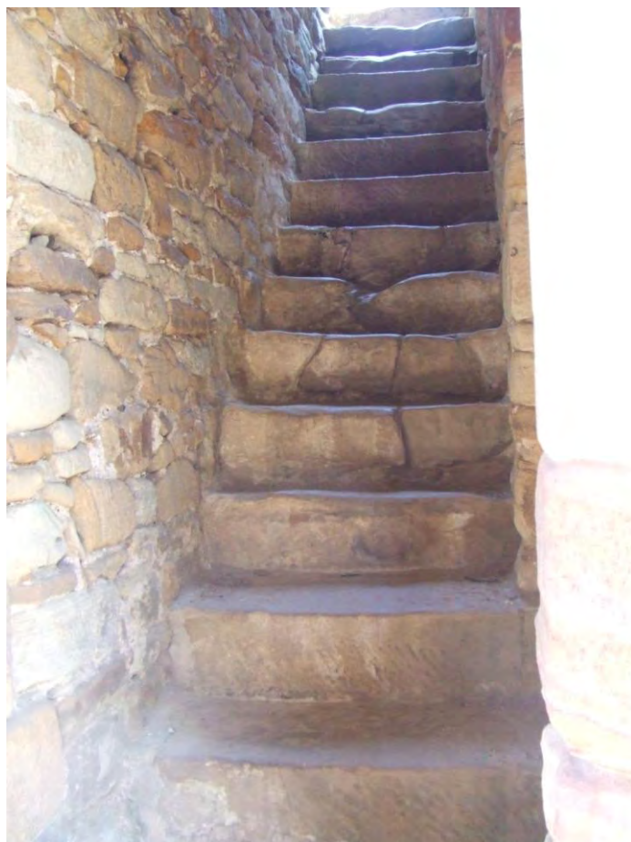
Figure 67. Ewloe Castle: Interior Stair. Illustrating the straight intramural stair in the Welsh Tower at Ewloe Castle. Photographer: C. Ryder.
