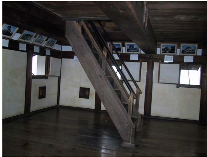
Figure 12. Kochi Castle: Interior Stair. Illustrating typical tenshu interior stairs. Photographer: E. Obershaw.
