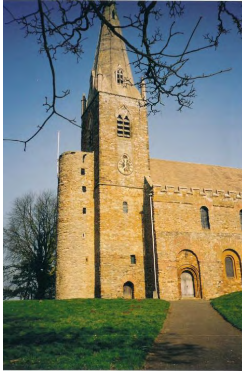
Figure 30. Brixworth Church. Illustrating the attached circular stair tower on the left. Photographer: C. Ryder.
