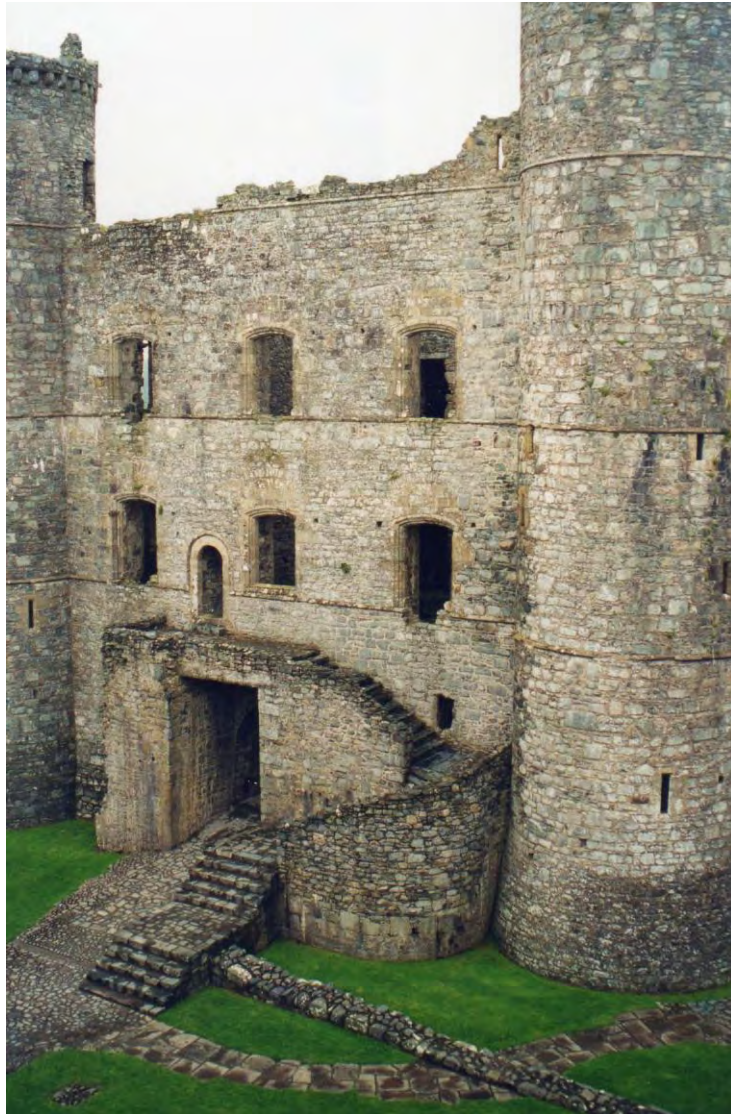
Figure 80. Harlech Castle: Rear of Gatehouse. Illustrating to the left and right extremes of the photograph the large stair towers. Photographer: C. Ryder.
