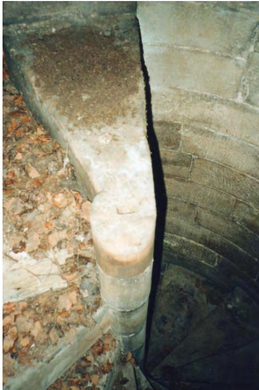
Figure 101. Nercwys, Tower: Top of the Spiral. Illustrating key-hole shaped stones with locating hole in the middle of the newel. Photographer: C. Ryder.
