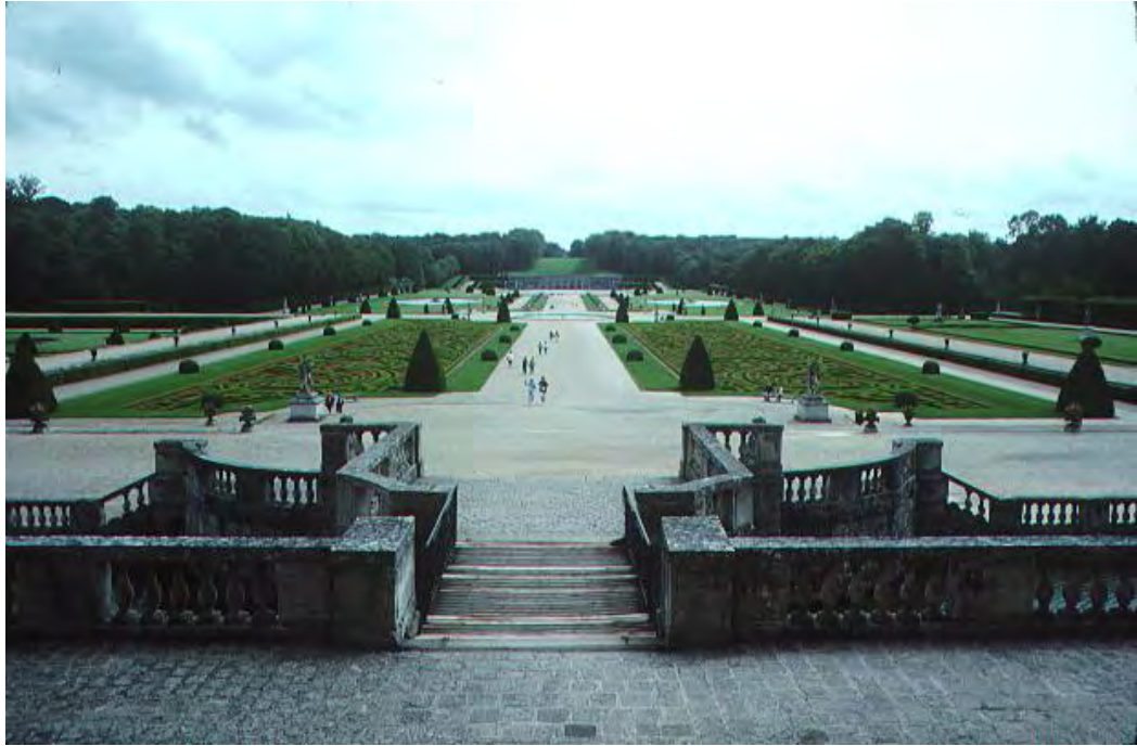
Figure 8. Vaux-le-Comte: Garden Stairs. Illustrating the steps with larger treads and low risers down to the garden. http://www.bc.edu/bc_org/avp/cas/fnart/arch/17thc/VauxleVicomte09.jpg .
