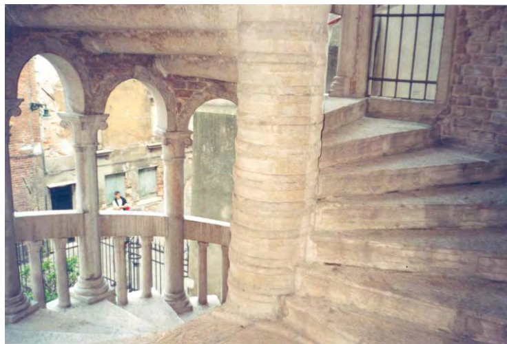
Figure 102. Venice, Bovolo Staircase. Illustrating the wide steps and broad newel and demonstrating how highly visibility user of the stair would be. Photographer: C. Ryder.
