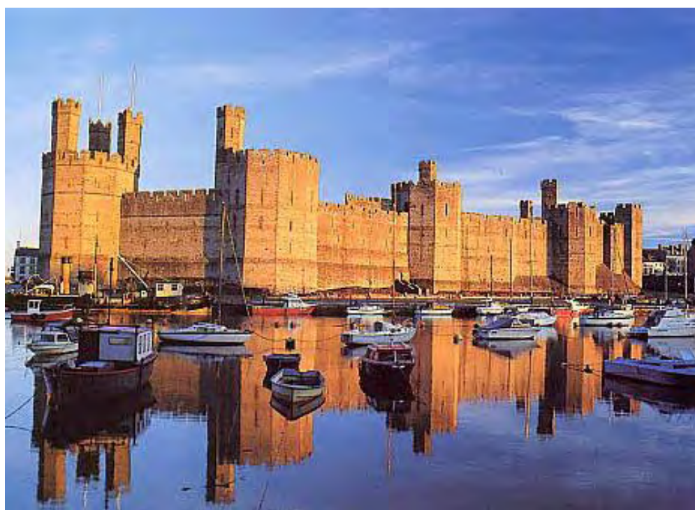
Figure 78. Caernarfon Castle. View from the south with the Eagle Tower on the left and the Queen's Tower on the right. http://www.busybus.co.uk/caernarfon-castle .
