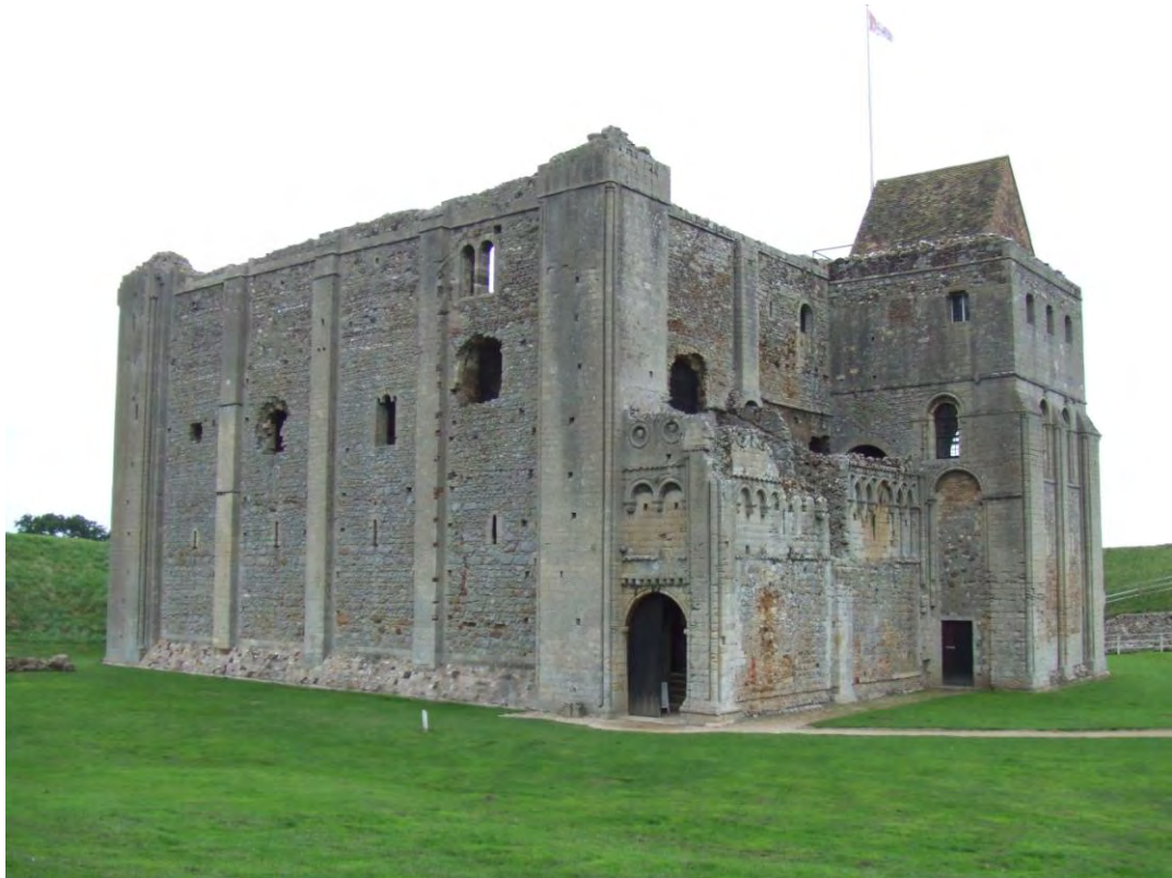
Figure 52. Castle Rising Keep and Forebuilding. Illustrating the entrance to the straight stairs in the forebuilding leading up to the Entrance Vestibule. Photographer: C. Ryder.
