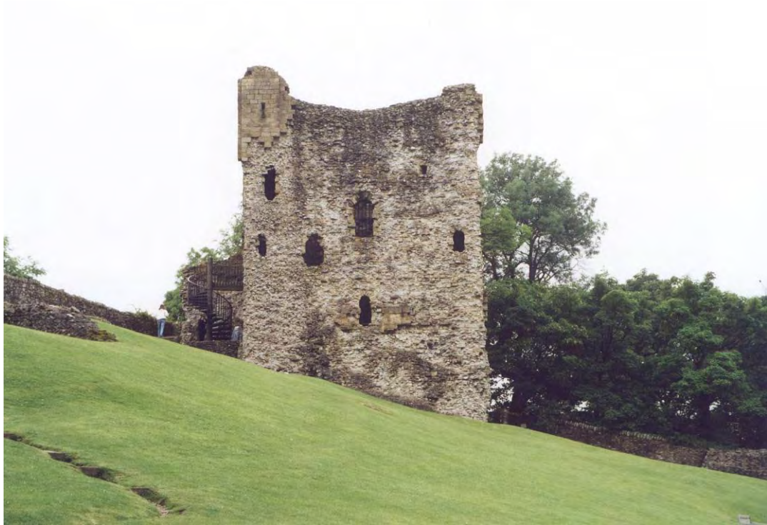
Figure 61. Peveril Castle Keep. Illustrating the slits lighting the spiral stair on the left and the larger widows on the diagonal. Photographer: C. Ryder.
