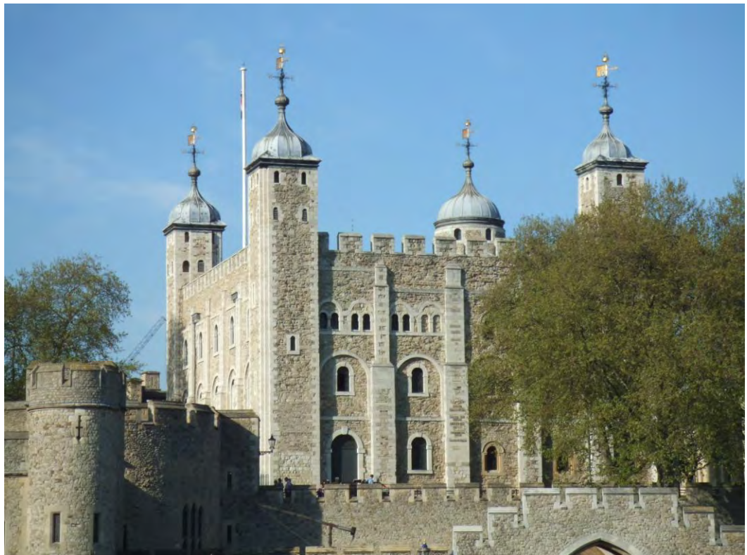
Figure 47. The White Tower. Illustrating the corner turrets containing the smaller spiral stairs. Photographer: C. Ryder.
