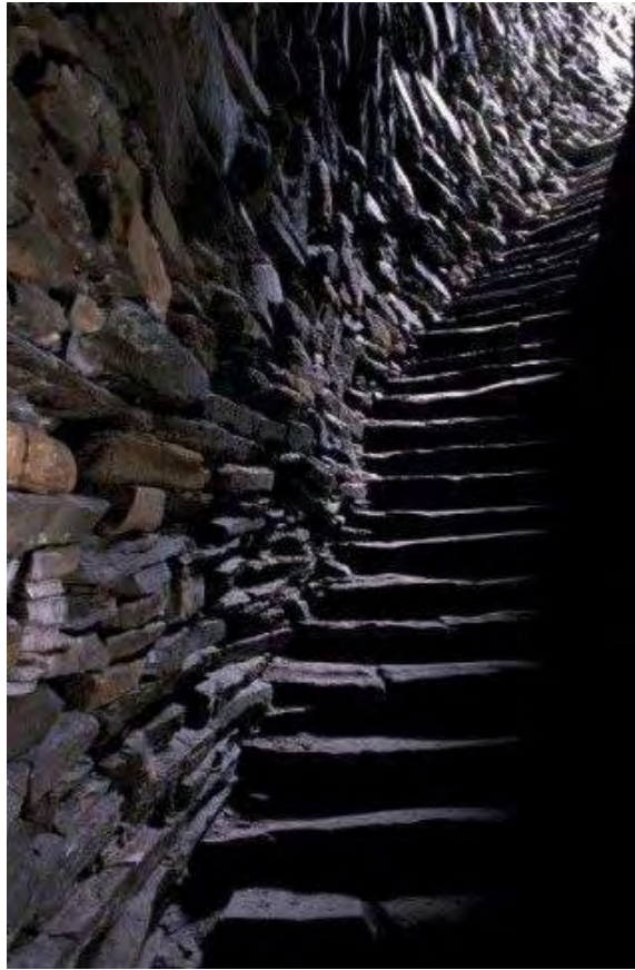
Figure 25. Shetland, Mousa Broch: Internal Stairs. Illustrating the form of the internal stair. Photographer: R. Harding.
