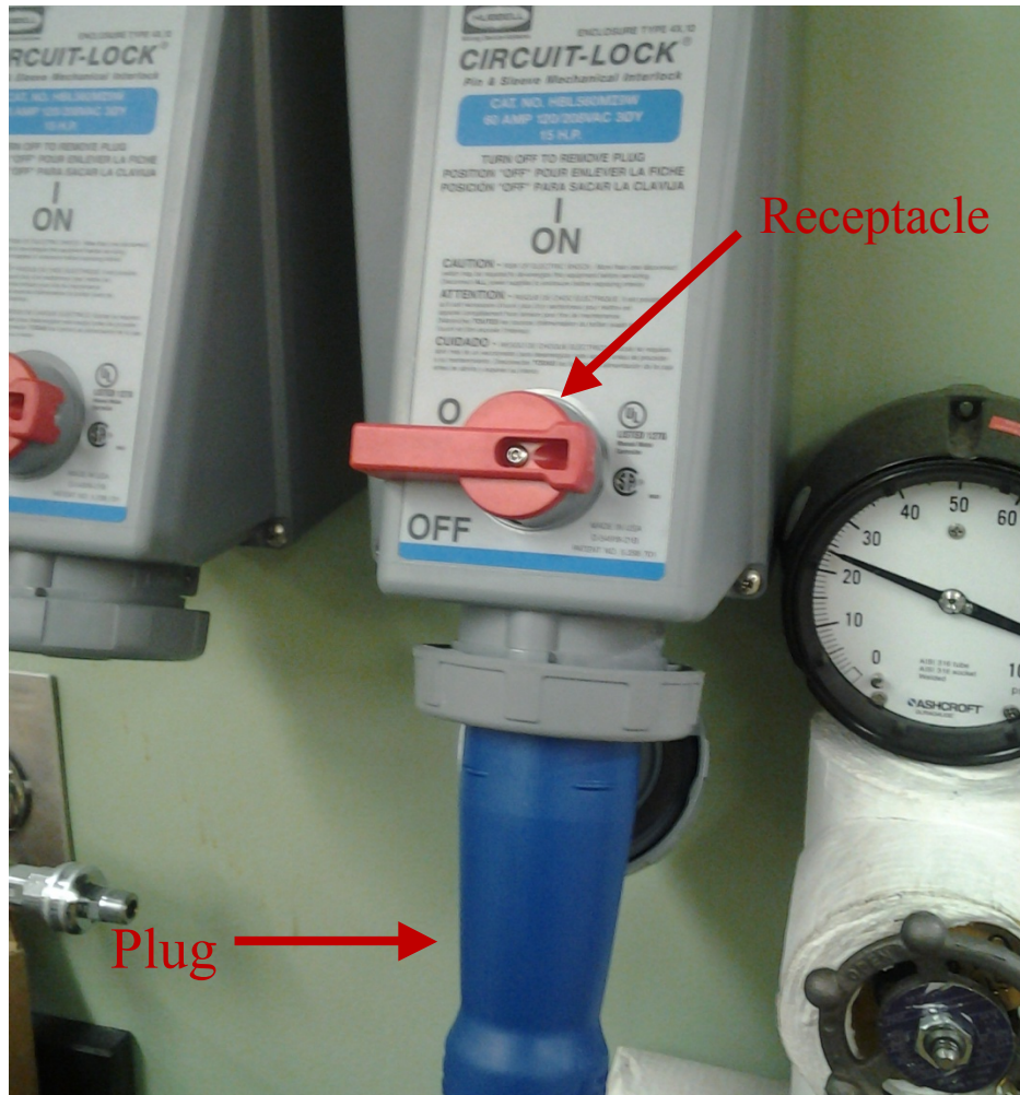
Fig 3-3: 240 VAC and 60 A plug and receptacle
