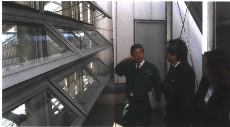
Figure 1-18: Wind obstruction (right side) installed near the exhaust openings of a Tokyo office building to ensure any wind-driven ventilation only contributes to the buoyancy-driven ventilation.
