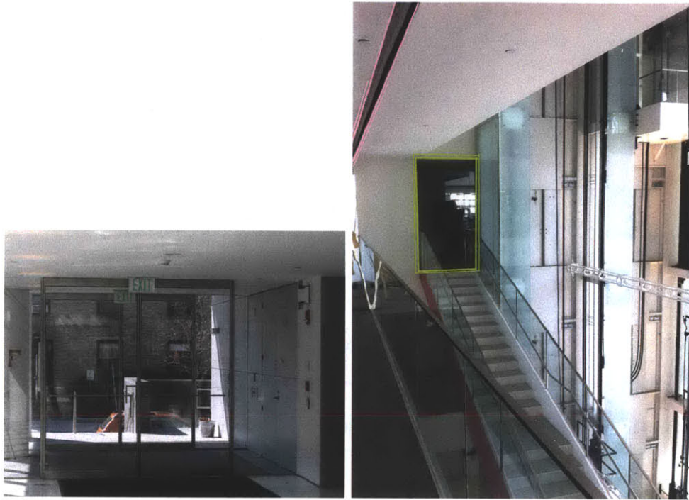
Figure 5-4: Photographs of the two openings into the atrium. (left) A single door on the ground floor is propped open during the experiment and (right) the third floor doorway outlined in green is left open. The fire door highlighted in pink along the ceiling (right) is closed during the experiment.
