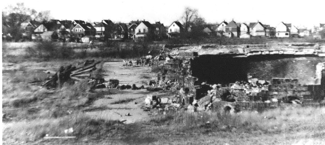
Figure 14. View of brick kilns from south side of selected site.
