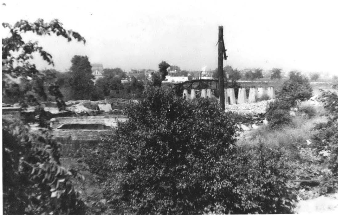
Figure 15. View of brick kilns from south side of selected site.
