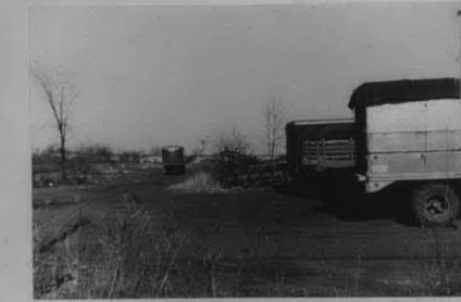
VIEW FROM SOUTHWEST CORNER
