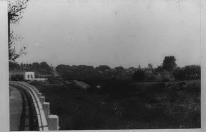
VIEW FROM NORTHEAST CORNER
