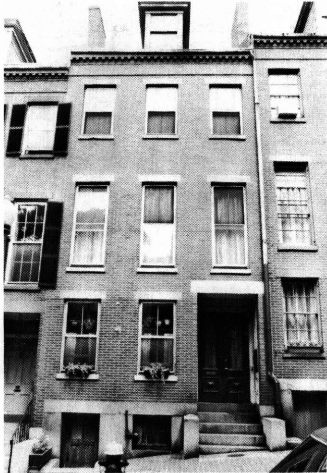
House on South Russell Street. Note the 3-part articulation of the facade, piano nobile, and basement entry.
