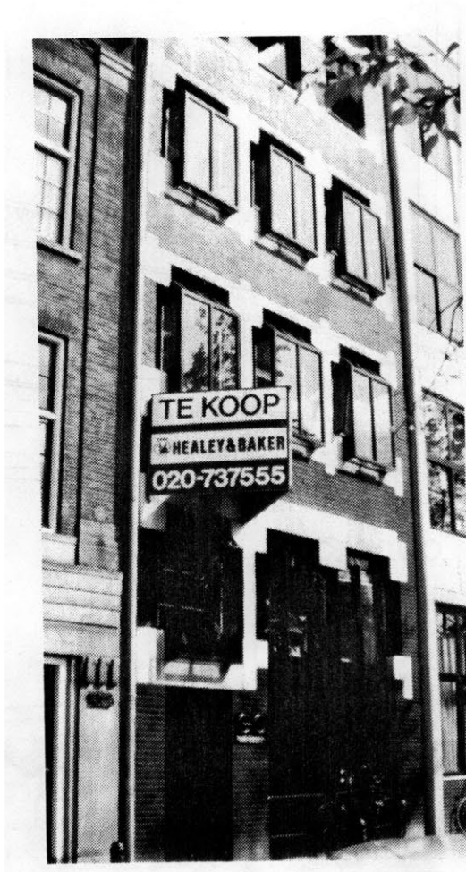
Window articulations in three-bay house in Amsterdam.
