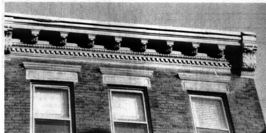
Cornice of building on Charles Street.
