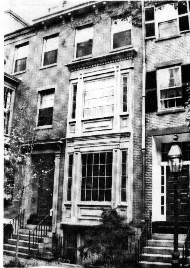
Aggregation of windows in Pinckney Street house occurs in a secondary material and different plane than brick wall surface.
