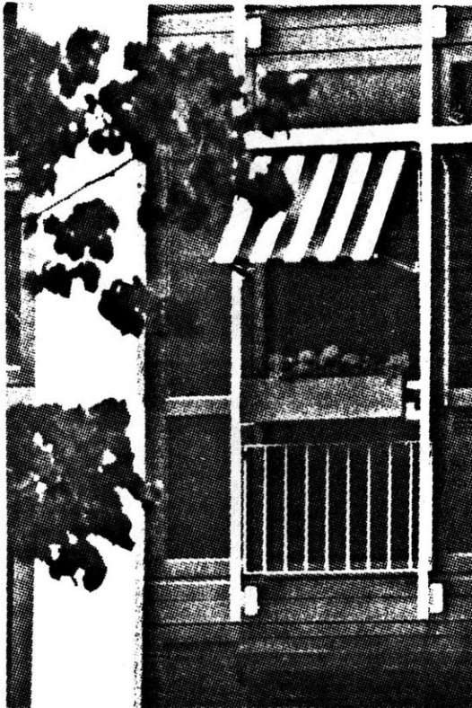
Metal framework around window holds flowers and awning. Project in Germany Gerd Eicher, Lothar Hetzig, and Franz-Jurgen Langer.
