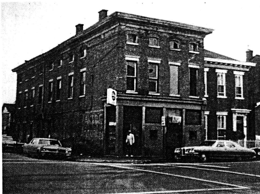
LARGER MULTI-UNIT BUILDINGS REINFORCED THE CORNER
