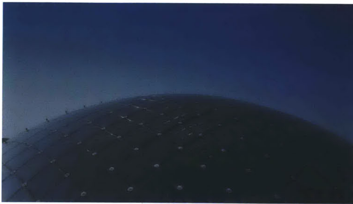
Figure 2.3 – External view of the Neckarsulm Swimming Arena.
