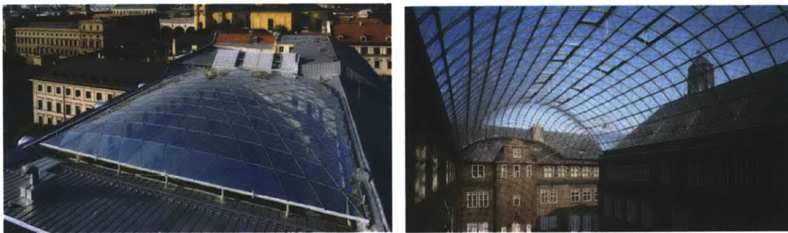
Figure 1.5 – Shallow shell at the Odeon in Munich (left); steeper shell at the Museum for Hamburg History (right).
