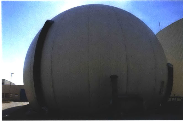
Figure 2.14 Gasholder for Biogas Produced from Sludge Digesters
