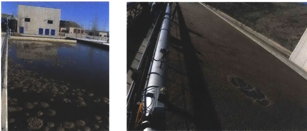
Figure 2.12 Secondary Biological Treatment process: Anaerobic Zone (left) and Aerobic Zone (right)
