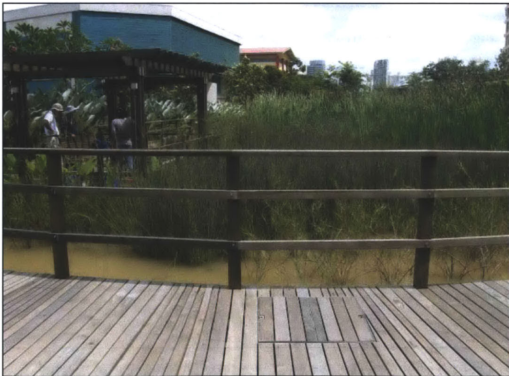
Figure 10 - Surface flow wetland (Photo: Laurie Kelldorfer)
