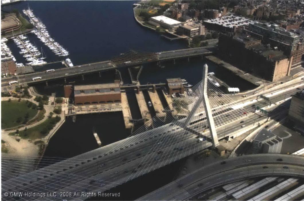
Figure 6. The new dam in 2008 (GMW Holdings LLC 2008)
