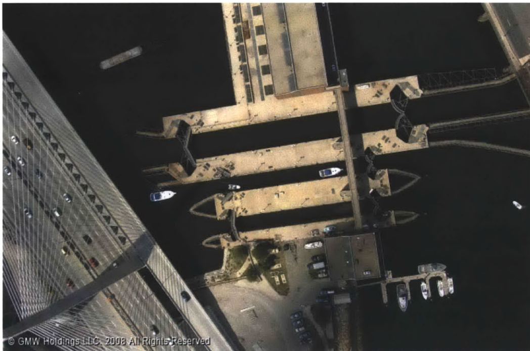
Figure 7. Locks on the new dam (GMW Holdings LLC 2008)
