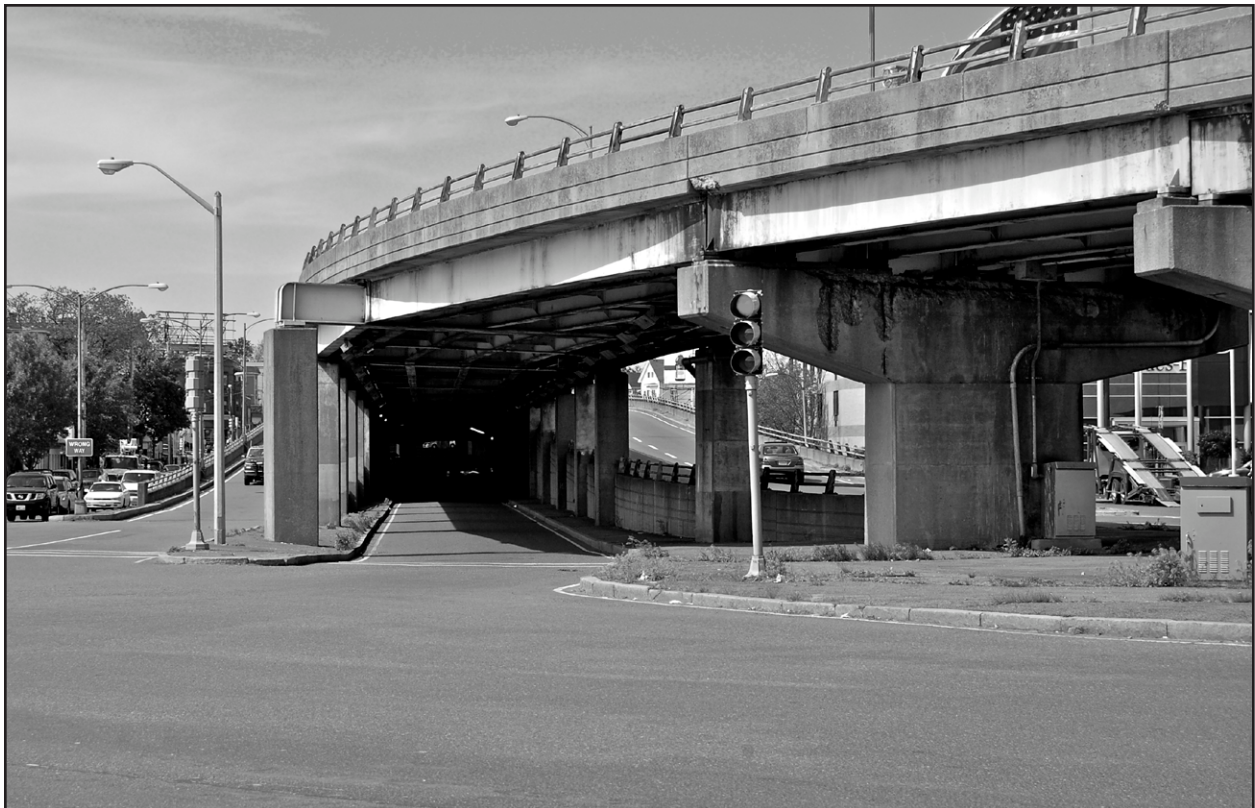
Figure 45: The northbound and southbound directions of McGrath Highway at Somerville are separated by the median in which the supports for the SB elevated sit (top) and also divided by the northbound tunnel (bottom).
