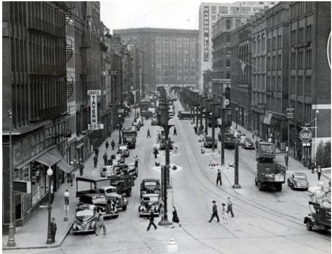
Figure 6: Atlantic Avenue Elevated before (top) and after demolition in 1942 (bottom)
