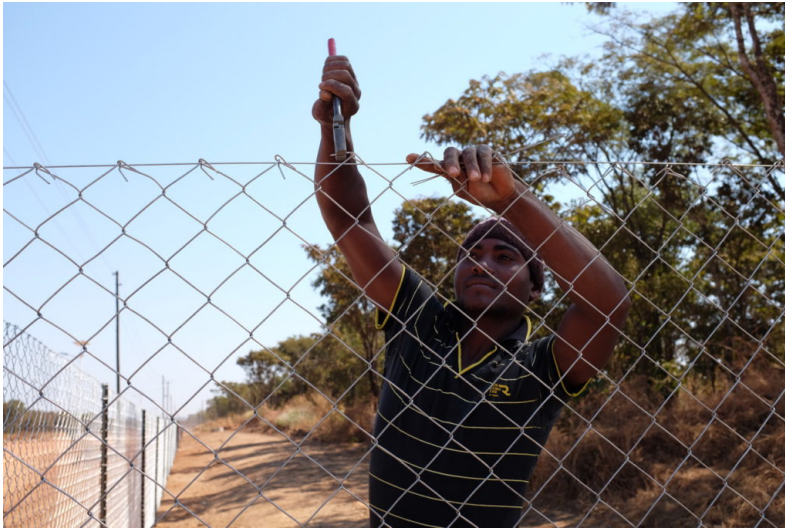
Worker constructing a fence within the Kabitaka premises
