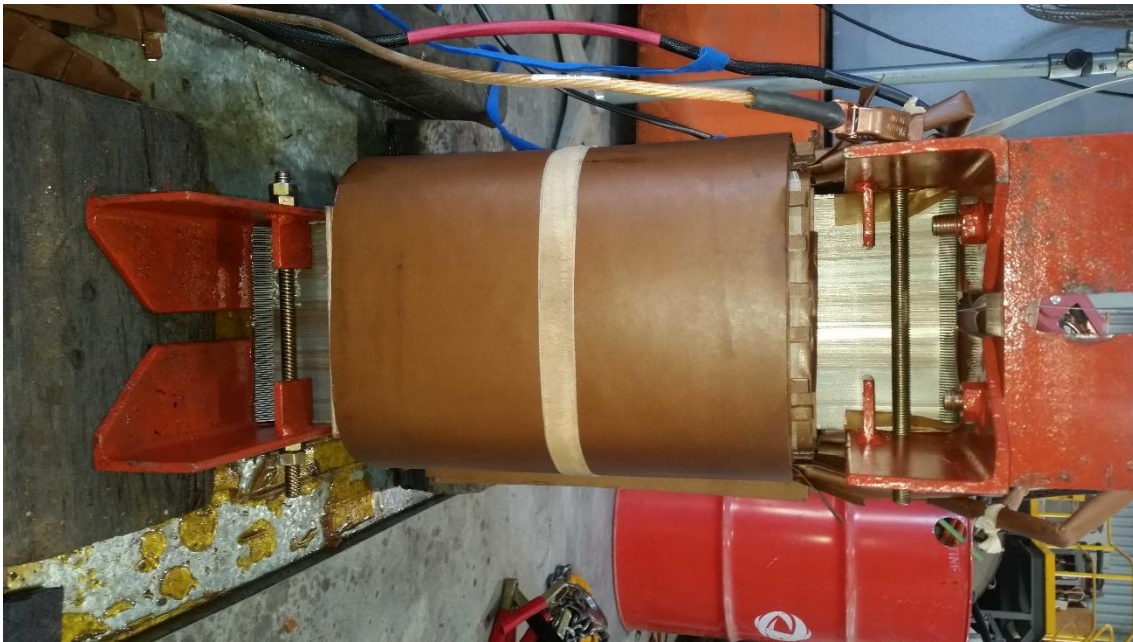
Figure 6.63 - East view of 90% windings axial displacement test iteration.
