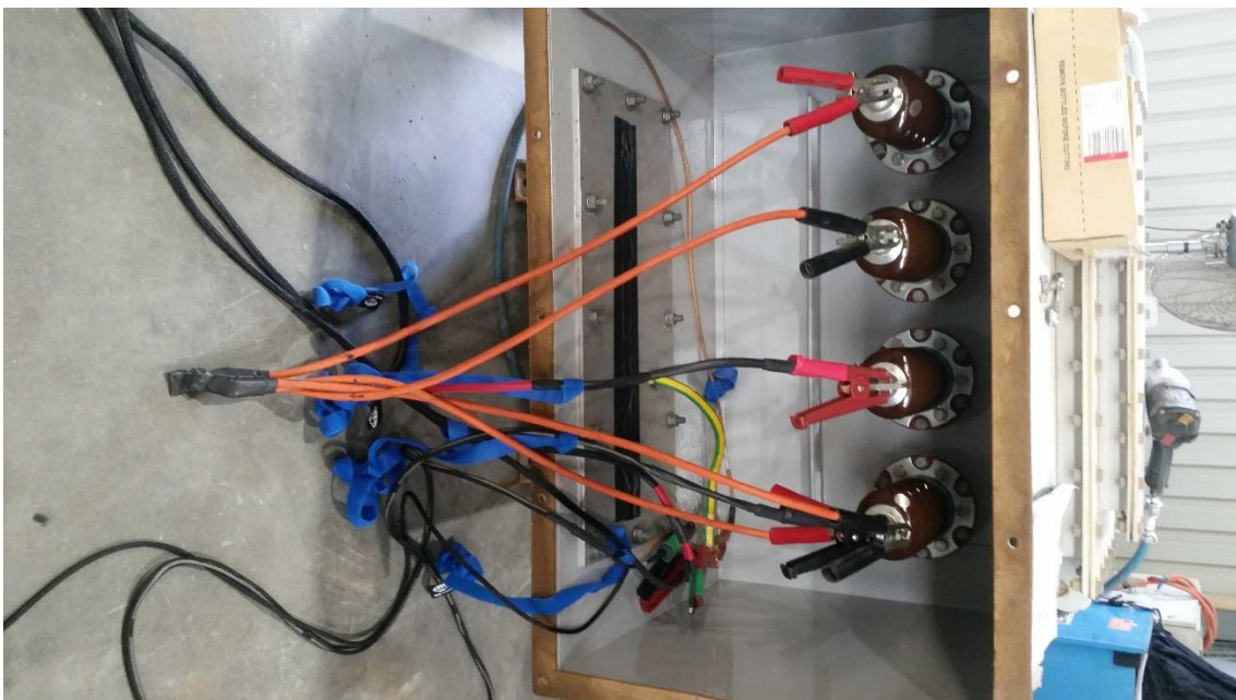
Figure 6.9 - Short circuit SFRA test set connection
