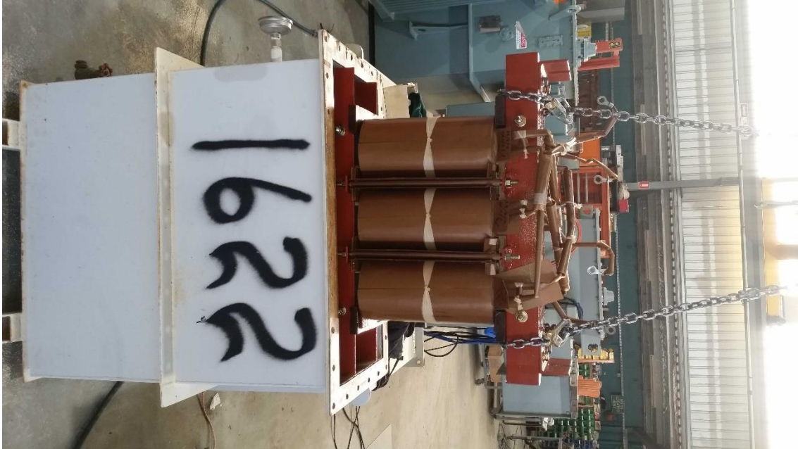
Figure 6.21 - Photo of the test earthing transformers core and coils being removed
