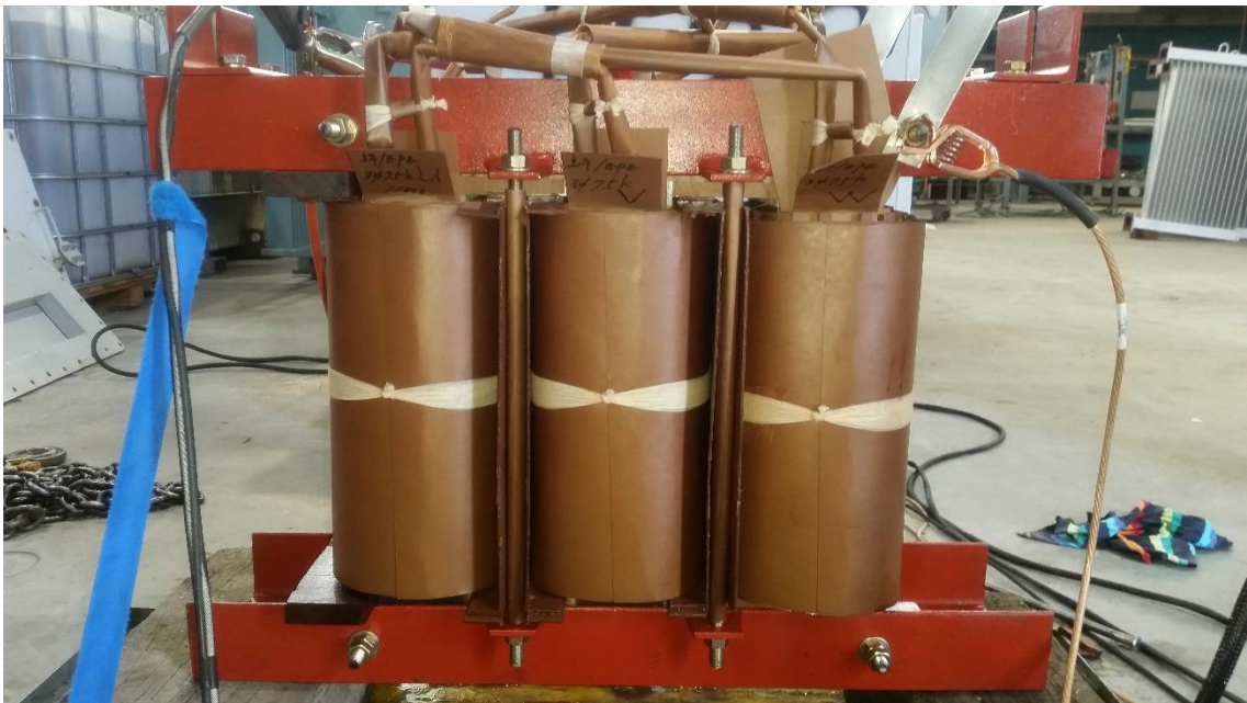
Figure 6.73 - North view of 45% windings axial displacement test iteration.
