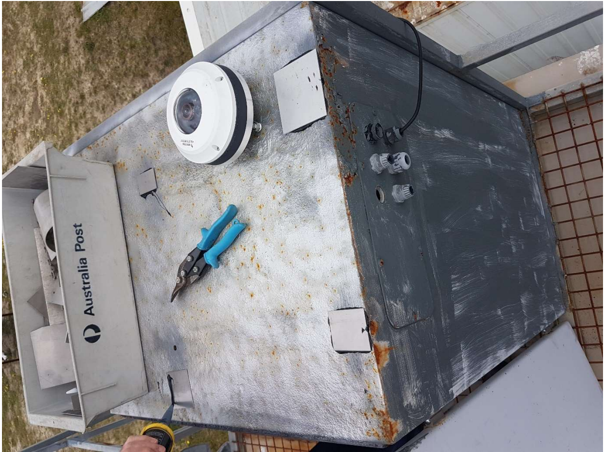
Figure 7 SkyCam_2 at REPS Facility Initial Mounting Design
