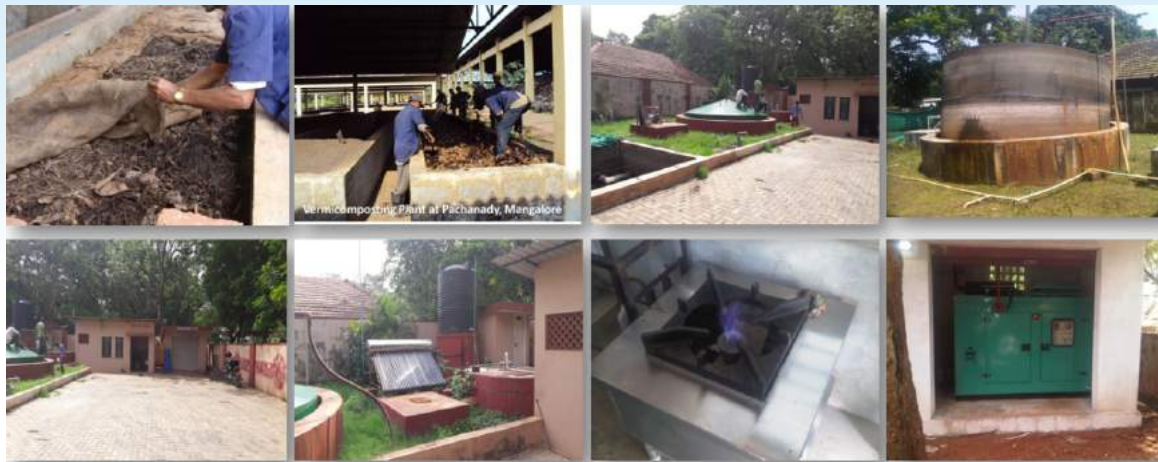
Vermi-composting process & Bio-methanation plant
