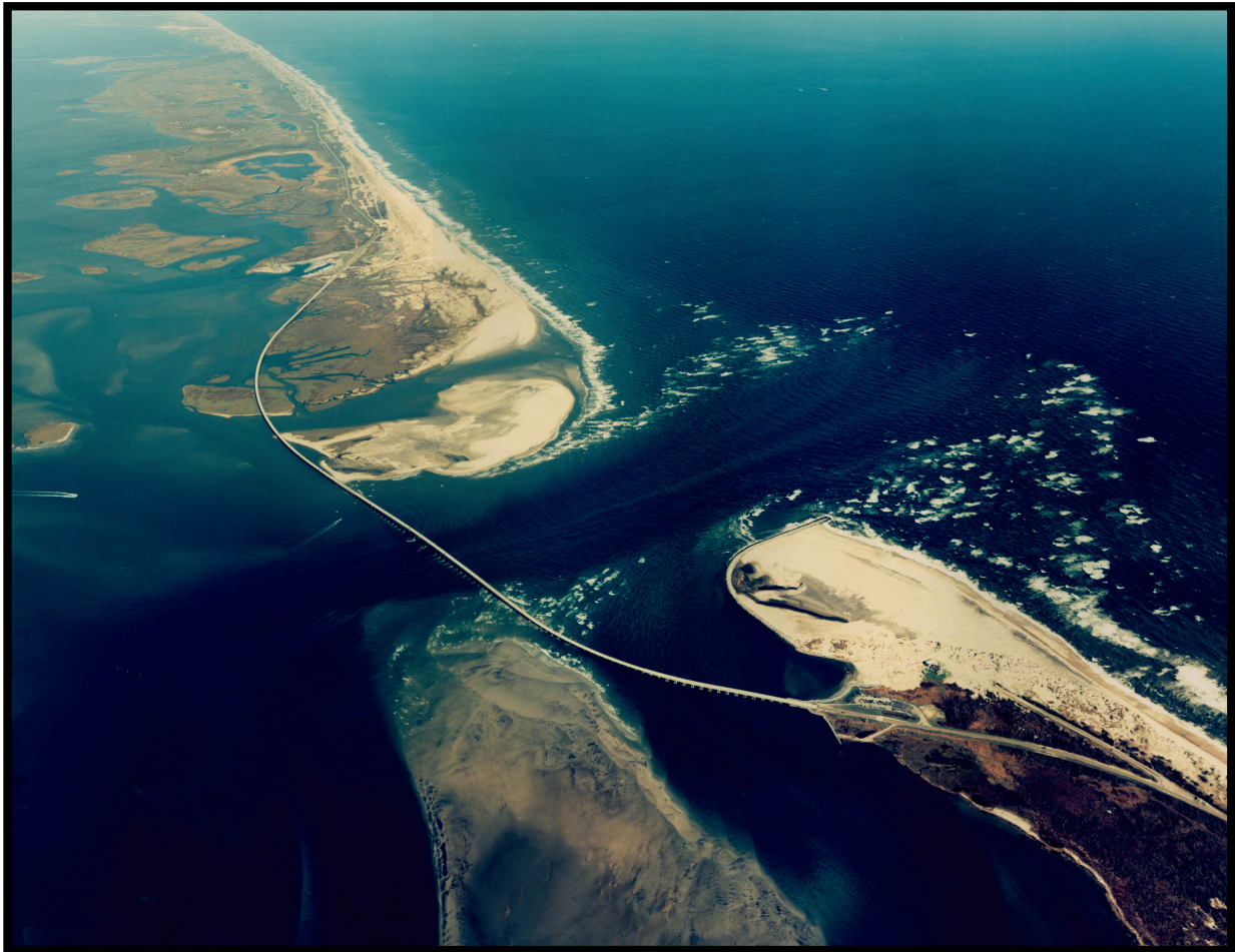
Figure 1.1 Aerial Image of Bonner Bridge looking North, 2008 (Photo by NCDOT)
