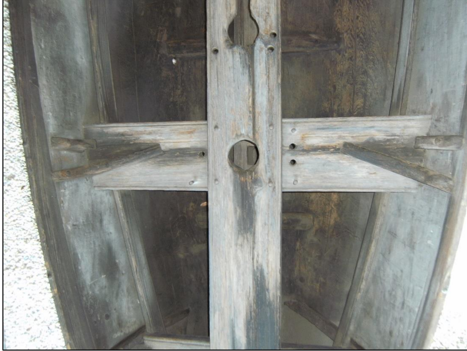
Figure 41: Thwart 2 and Surrounding Structures from Above (photo by author 2012)
