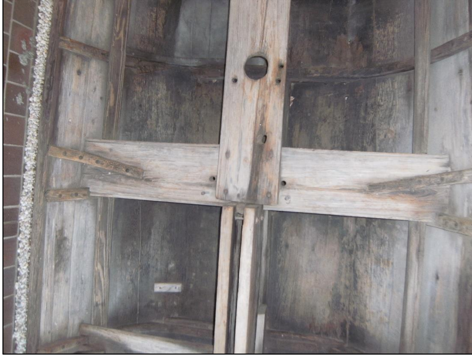
Figure 45: Thwart 6 and Surrounding Structures from Above (photo by author 2012)
