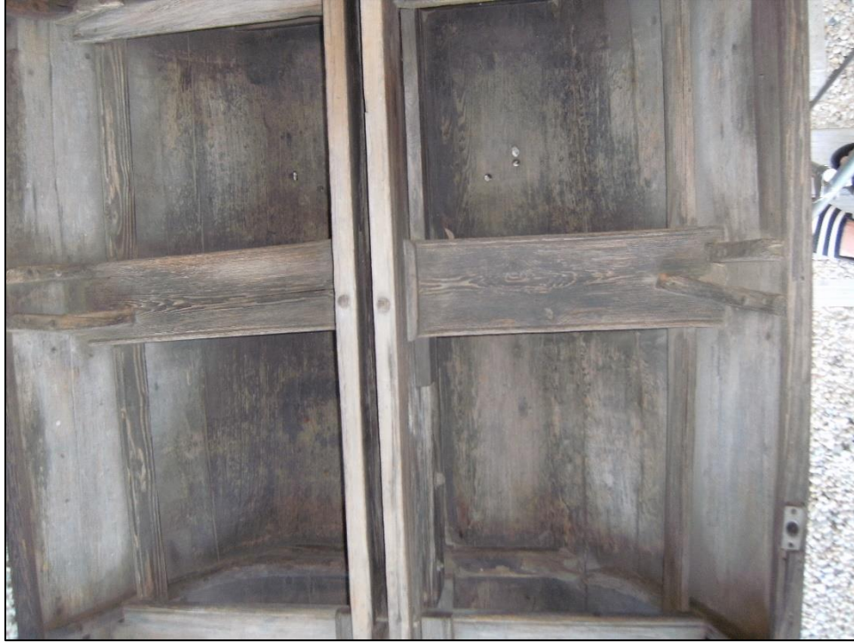
Figure 43: Thwart 4 and Surrounding Structures from Above (photo by author 2012)
