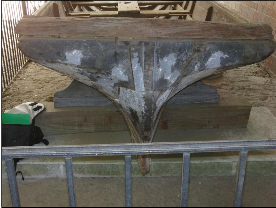
Figure 29: Bessie Transom with Various Repairs (photo by author 2012)
