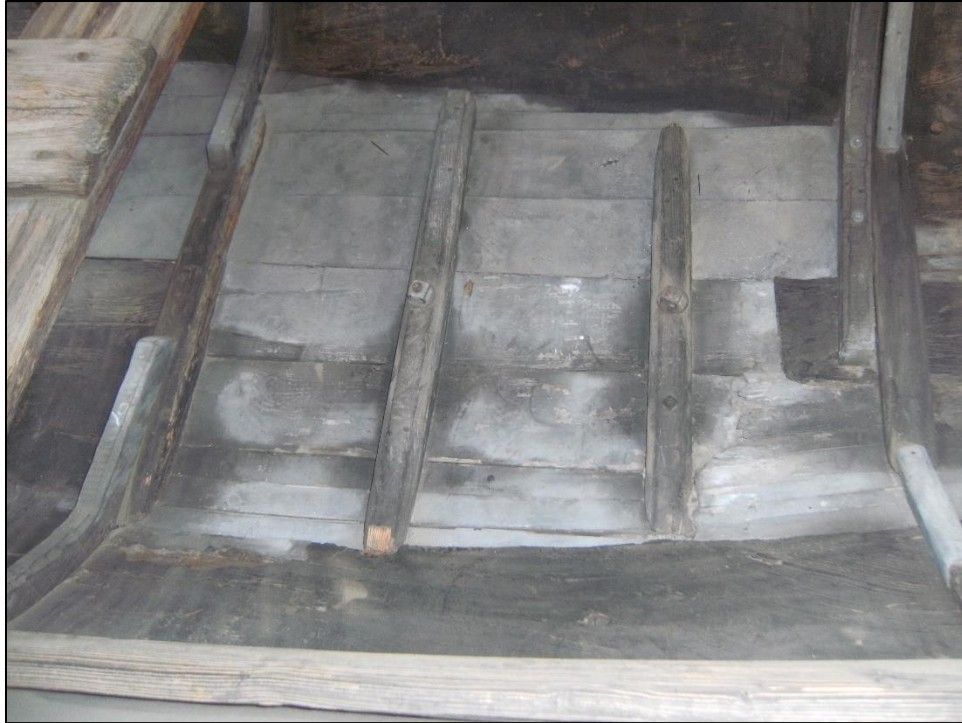
Figure 47: Stern Repair Area from Port Side (photo by author 2013)
