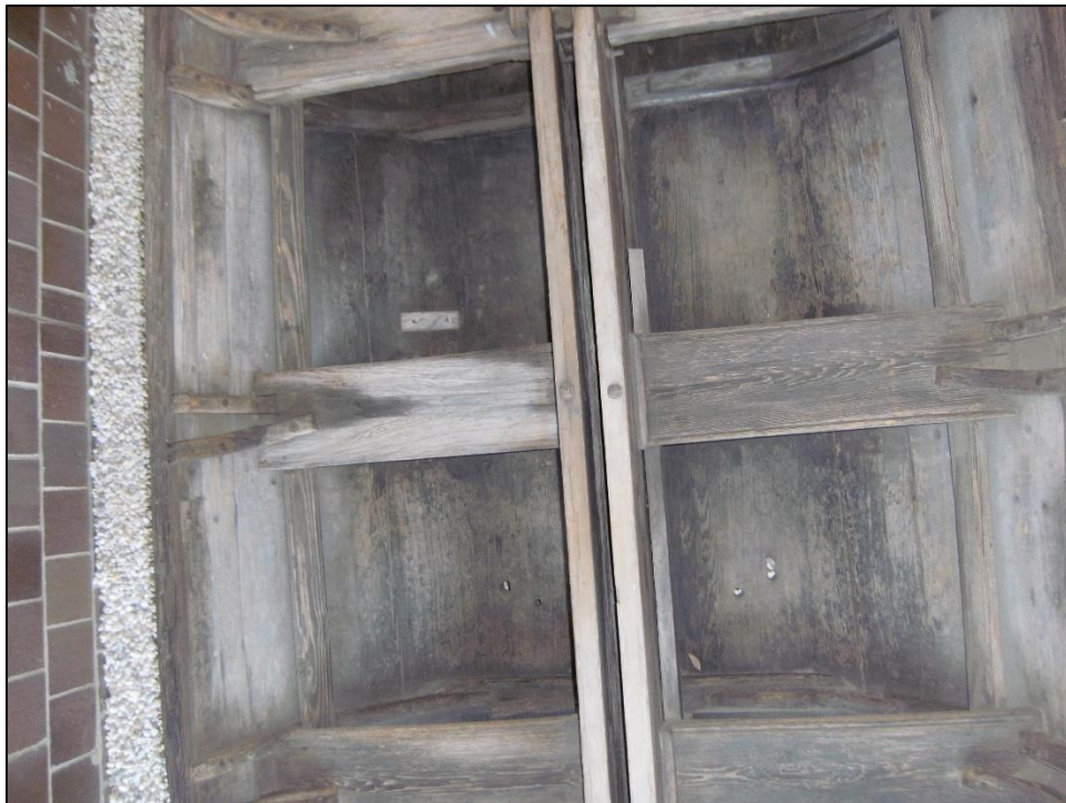
Figure 44: Thwart 5 and Surrounding Structures from Above (photo by author 2012)
