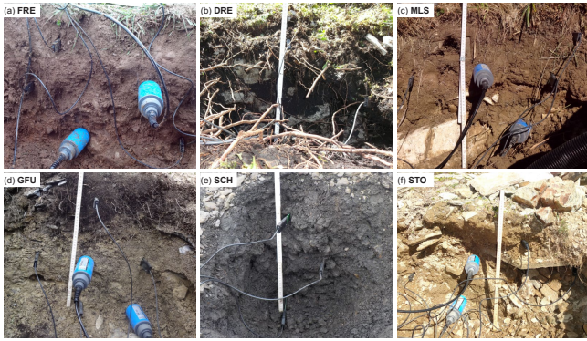
Figure 3. Illustration of the soil characteristics and sensor installation for all SOMOMOUNT stations.
