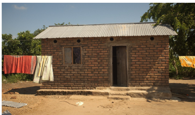
Figure 5. Front view of house B after installation of the eave tubes. The bedroom is on the left.
