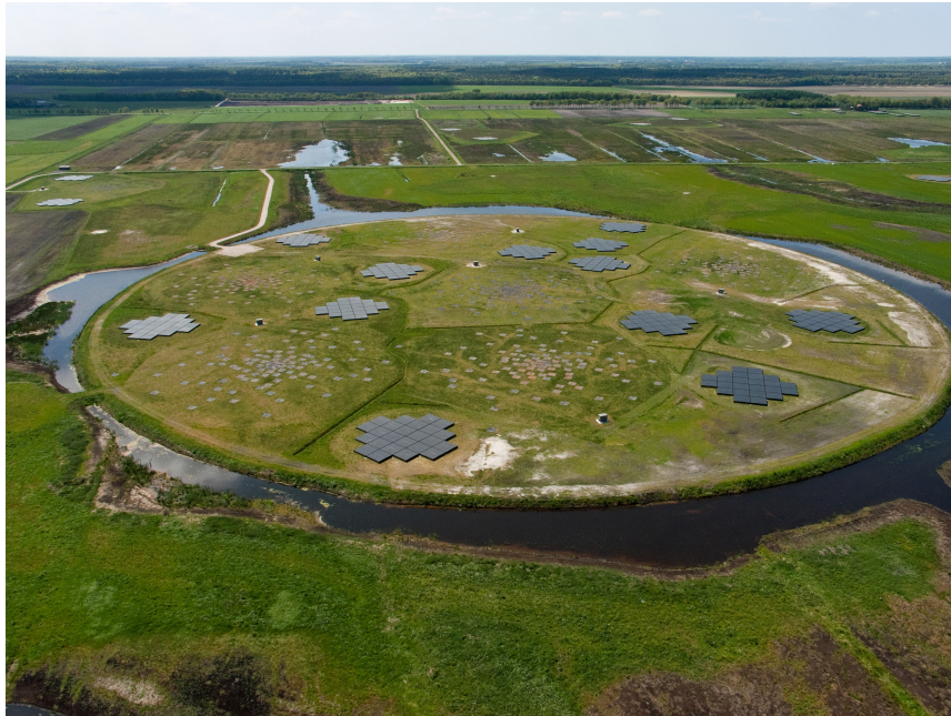
FIGURE 1.1: Image of the LOFAR ‘superterp’, where the 6 central stations of the array are located. The small black squares are HBA tiles containing 16 antennas. Image credit: LOFAR / ASTRON.
