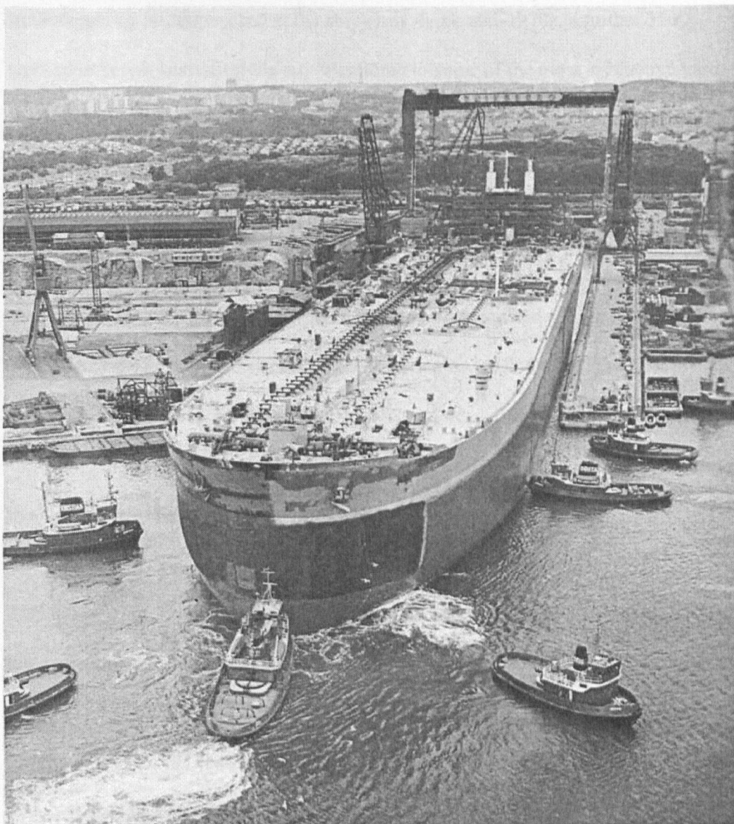
Plate 4a: The 402,000DWT T/T Nai Genova, one of the very last ships to be finished at the Eriksberg shipyard, pictured here being launched in 1978. Source: Gothenburg Shipbuilding Historical Society
