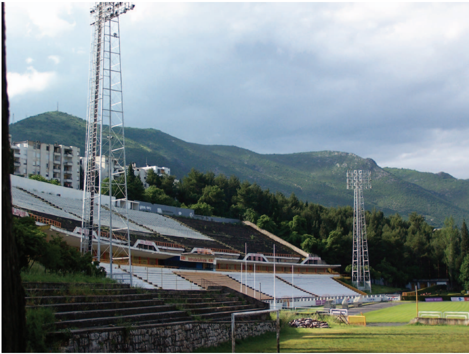
FIGURE 5. THE DILAPIDATED BIJELI BRIJEG STADIUM IN WEST MOSTAR
