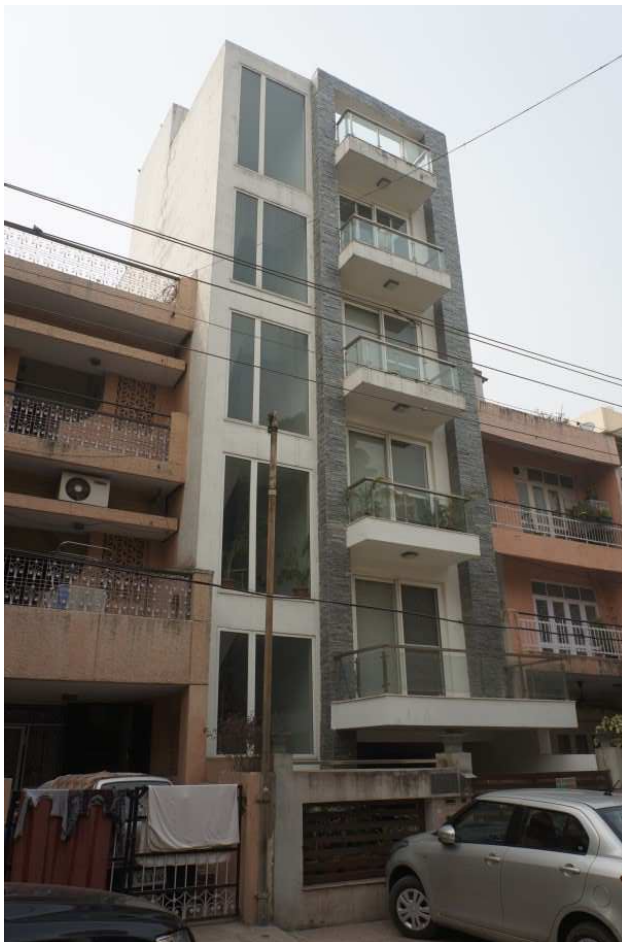
Figure 2.4: Newly Rebuilt House in the South Delhi Neighbourhood Safdarjung Enclave. Photo: Annika Mayer
