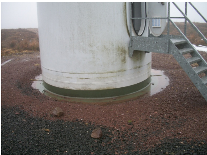
Figure 4: EMBEDDED CAN, TOWER AND FOUNDATION
