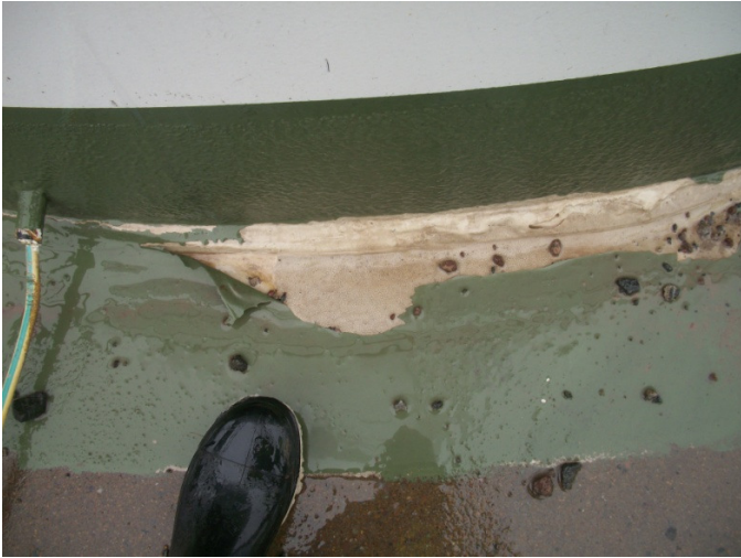
Figure 7: WATERPROOFING DETERIORATION
