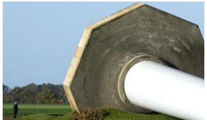
Figure 2: GOLDENSTEDT WIND TURBINE COLLAPSE
