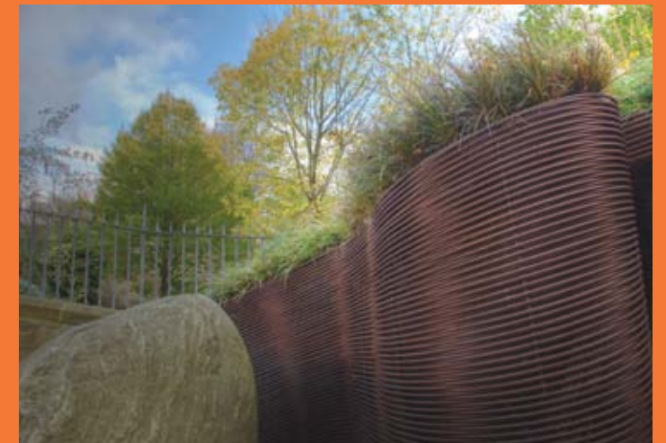
Right: Detail view of completed Composting Shed Edinburgh in Collaboration with Nicholas Groves-raines
