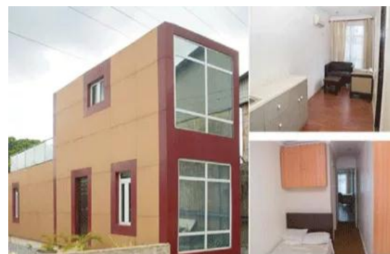
Figure 2: A shipping container building in Nigeria
