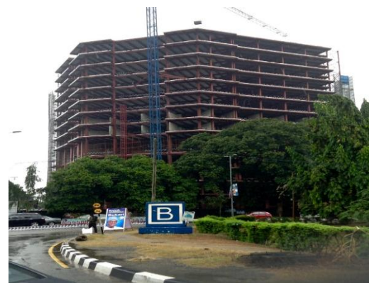
Figure 1: Steel and Concrete composite construction in Lagos State, Nigeria
