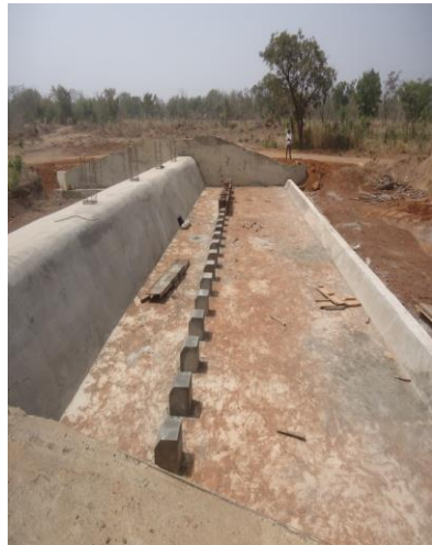
Figure12 Spillway under construction
