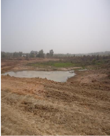
Figure 13 Seepage from original dam
