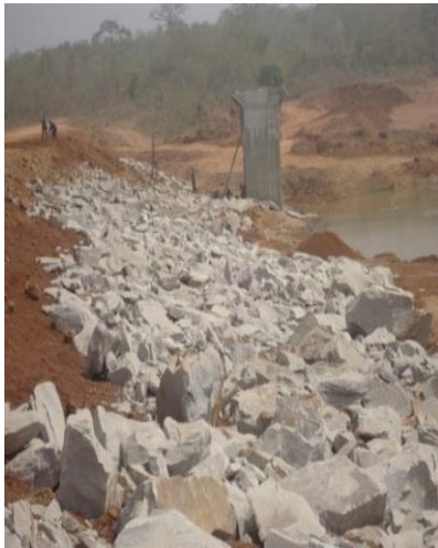
Figure 11 Re-construction in process
