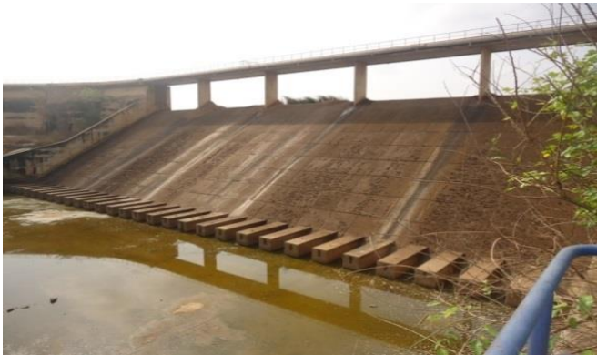
Figure 16 Spillway showing freeboard
