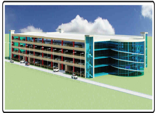
Figure 3 Right side view showing the external ramp
