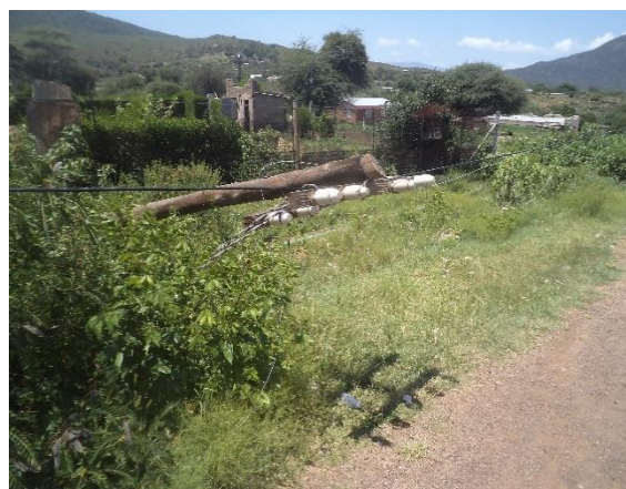
Figure 5.3: Vandalised telecommunication infrastructures in Ga-Malekane village.
