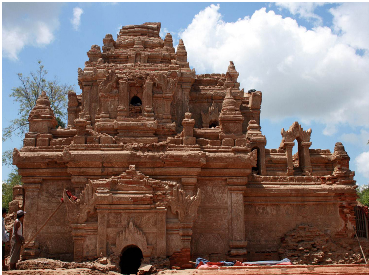
Fig. 12.4: East façade Ta Mok in 2010 (Photo: Sithu, Ta Mok Project).
