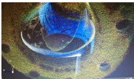
Figure 8. a 3D visual of corrosion in a CAD package, nodes of accretion and wear pattern is observable
