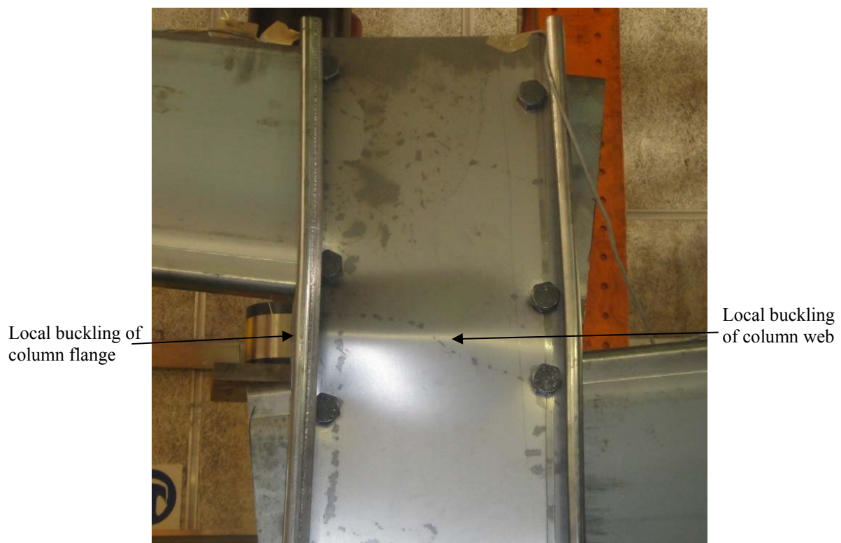
Figure 11: Local buckling failure in ECT-1 frames
