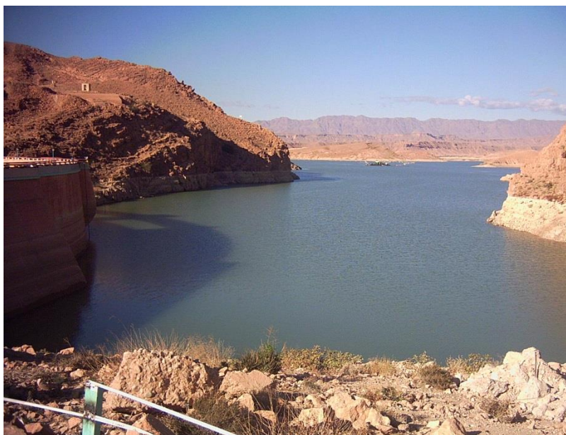
Fig. 3 Overview of Foum El Gherza dam (Remini, 2004)
