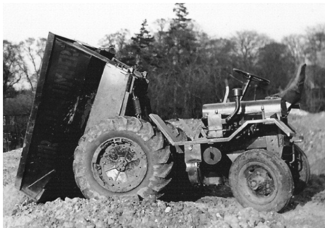
Obr. 2.1 Dumper – firma E.Boydell [12]
