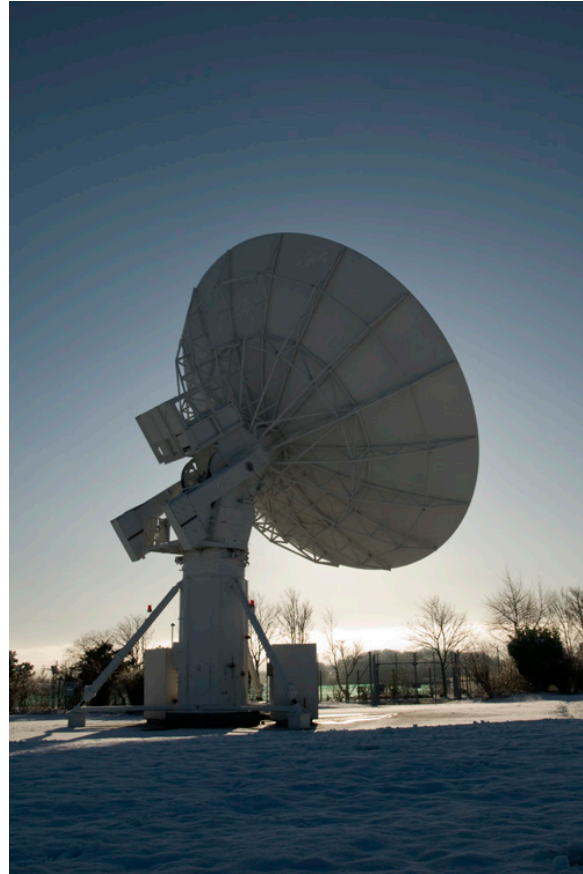
Figure 29 – 12 m antenna dish at Rutherford Appleton Laboratory in the UK with the potential of becoming an X-band ground station
