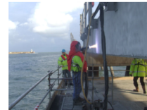
Figure 1 Photograph Showing Application of a Thermal Spray Coating to a Concrete Structure
