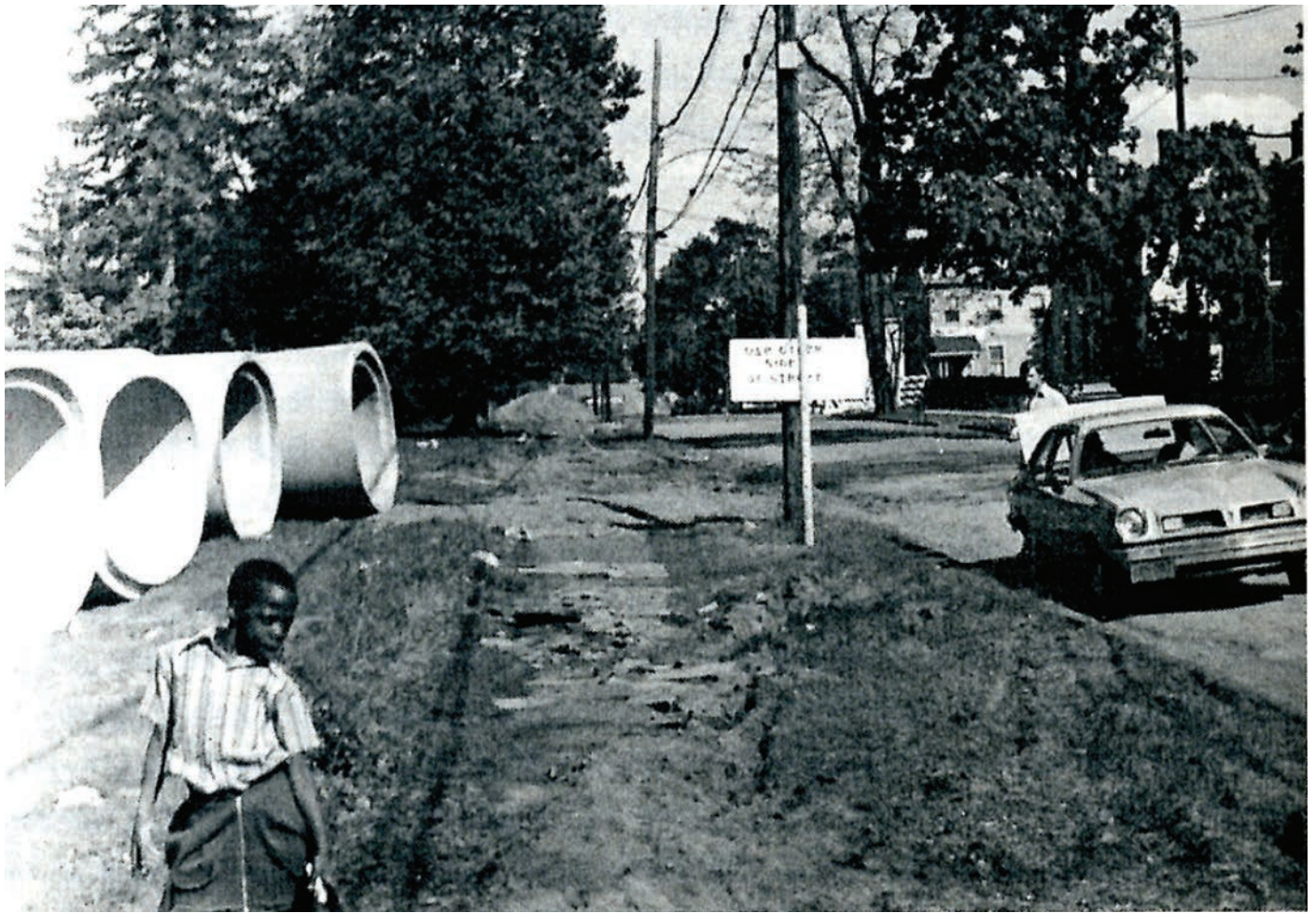
The Arterial under construction, 1977. Image from Flad and Griffen, 212.
