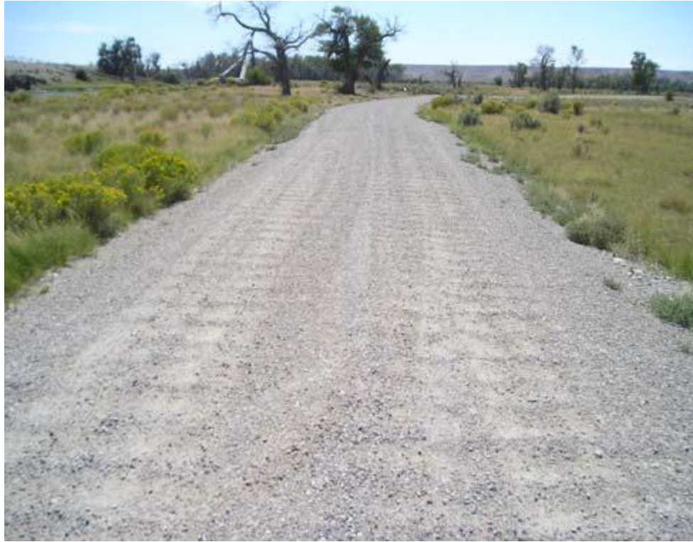
Figure 1-6: Washboarding on unpaved roads in Seedskaadee NWR [Woll et al, 2008].
