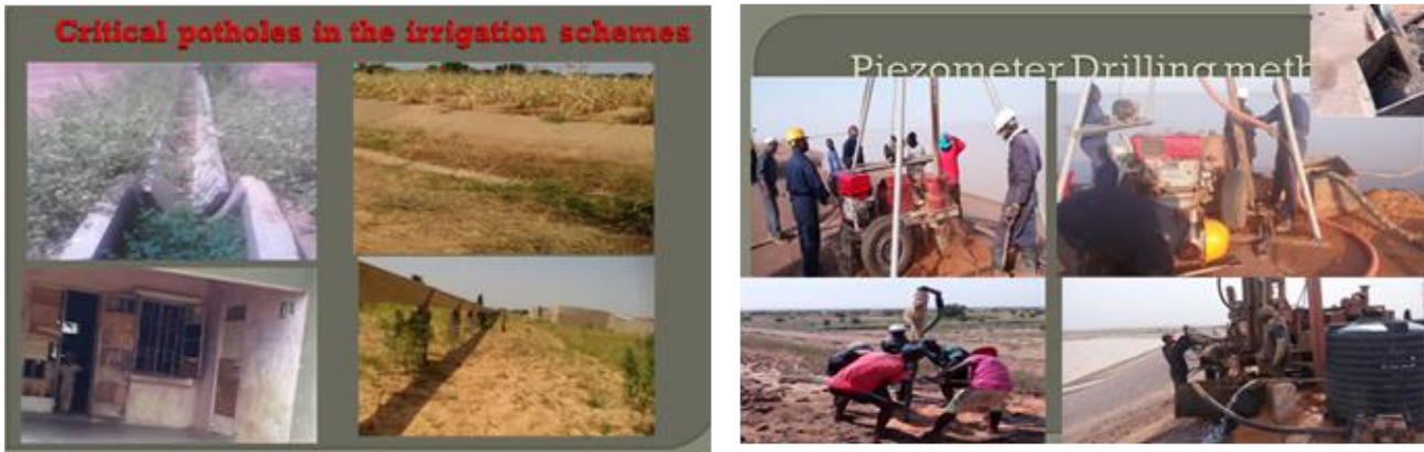
Figure 2: Poorly maintained canals and accommodation at the Project areas (left); Drilling at the dam (right)
